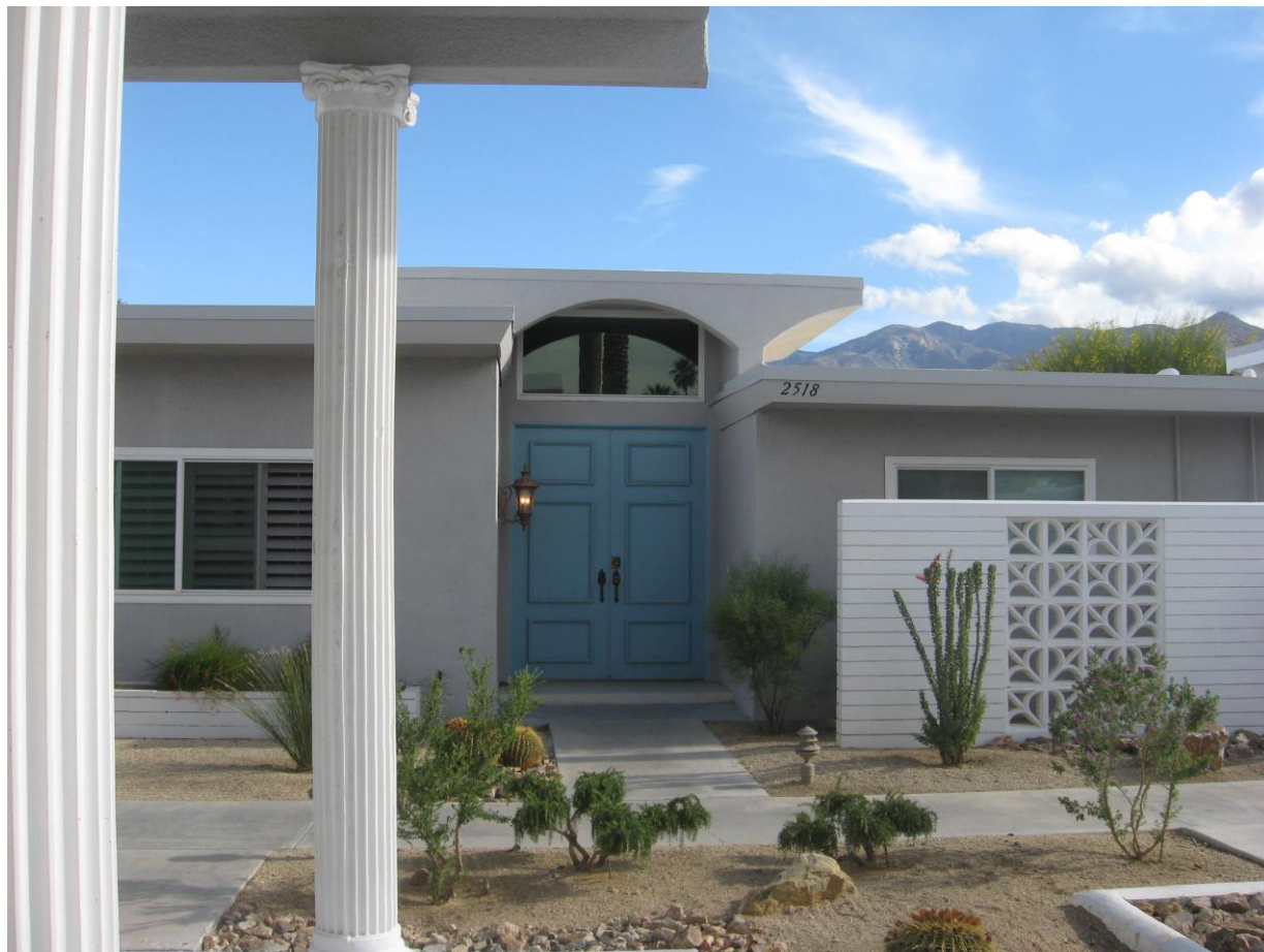
Villa Roma unit showing raised “platform” style of roof above entry. Note eaves, variegated roof heights, recessed entry, clerestory windows, carriage entry light and “Sprite” screen block wall, all typical original design features. Windows are vinyl-type replacements.
