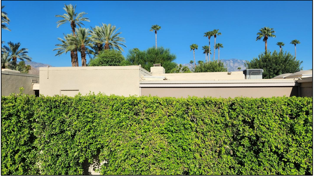
Looking due west from an elevated position in the east Tamarisk Gardens parking lot is the roof of Tamarisk Gardens #5. The rooftop air-conditioning unit, skylight, and fireplace chimney can be seen.
