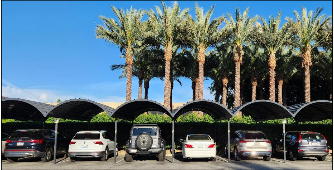
Looking due east towards the Tamarisk Country Club is one of Tamarisk Gardens' barrel-roofed parking structures.
