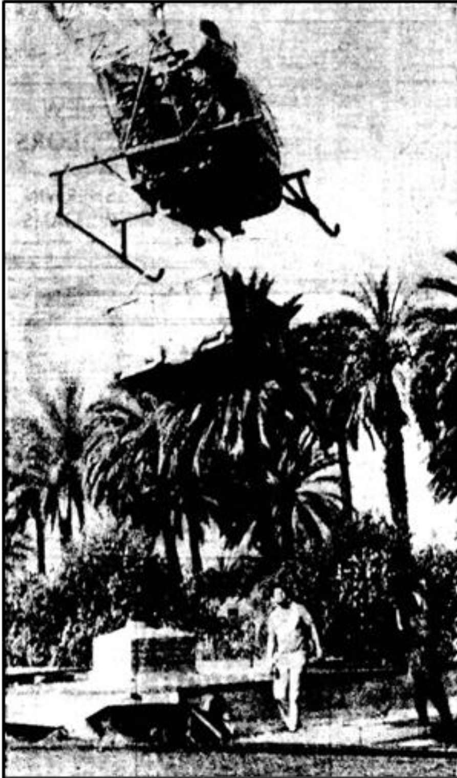
The May 7, 1965 issue of the Desert Sun newspaper showed this photograph captioned "WHIRLYBIRDS were used this week to place air conditioners atop the Tamarisk Gardens homes under construction on Wonder Palms Road near Highway 111. The action photo at top was made as Pilot Don Landell lowered one of the units into position, an operation which took an average of a minute and a half per unit for the entire job."
