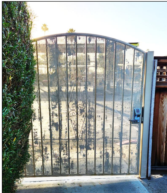
At the far northeast corner of the Tamarisk Gardens complex is a substantial metal gate allowing pedestrian and golf cart access to the adjacent Tamarisk Country Club. A number of gates between the two complexes remain intact.
