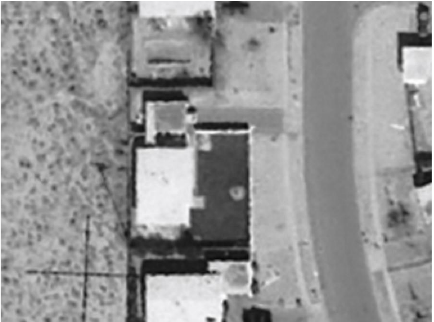
This 1965 aerial photograph shows the configuration of the plywood fence enclosing the grassy front yard area. Courtesy Geospatial Collection, UCSB Library, University of California, Santa Barbara.
