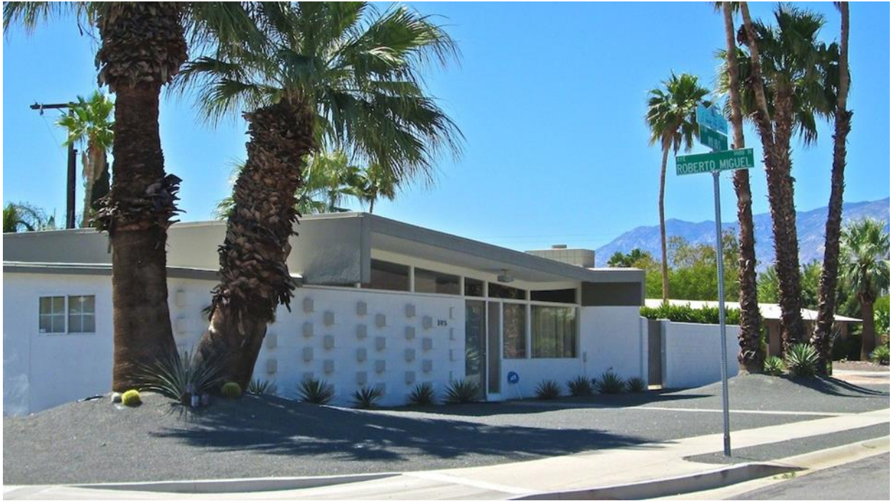
Architects Wexler and Harrison at El Rancho Vista Estates devised some inventive shadow block patterns.
