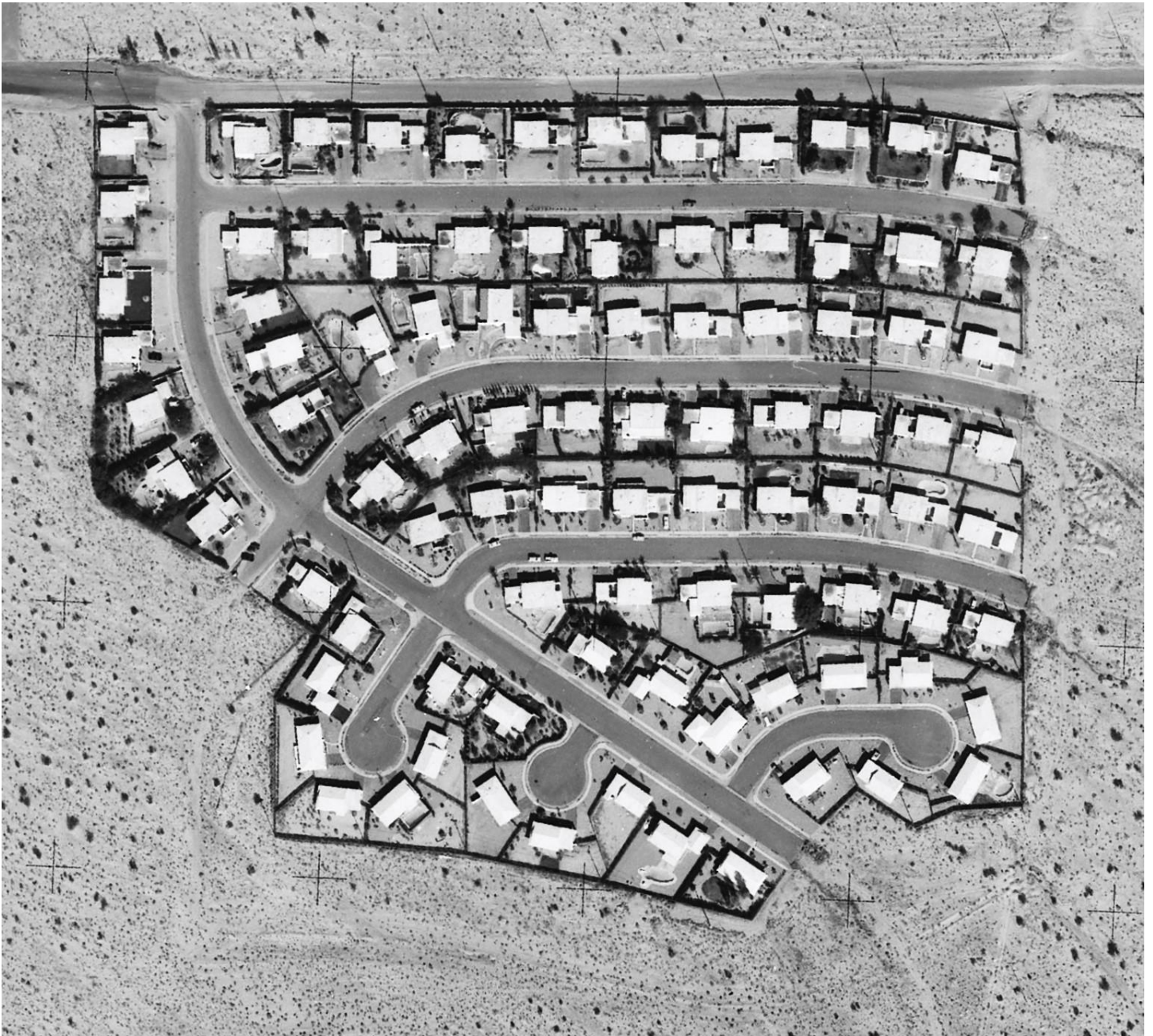
A 1965 aerial photo shows both the 1960-1961 Wexler and Harrison-designed houses, as well as the non-Wexler and Harrison houses from 1961-62, grouped more toward the bottom of the photo. Courtesy Geospatial Collection, UCSB Library, University of California, Santa Barbara.
