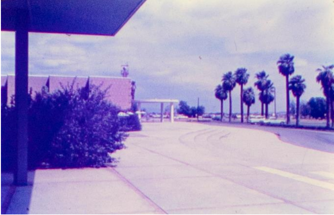
The “Modular Garden” in front of the Primary Façade – East.
