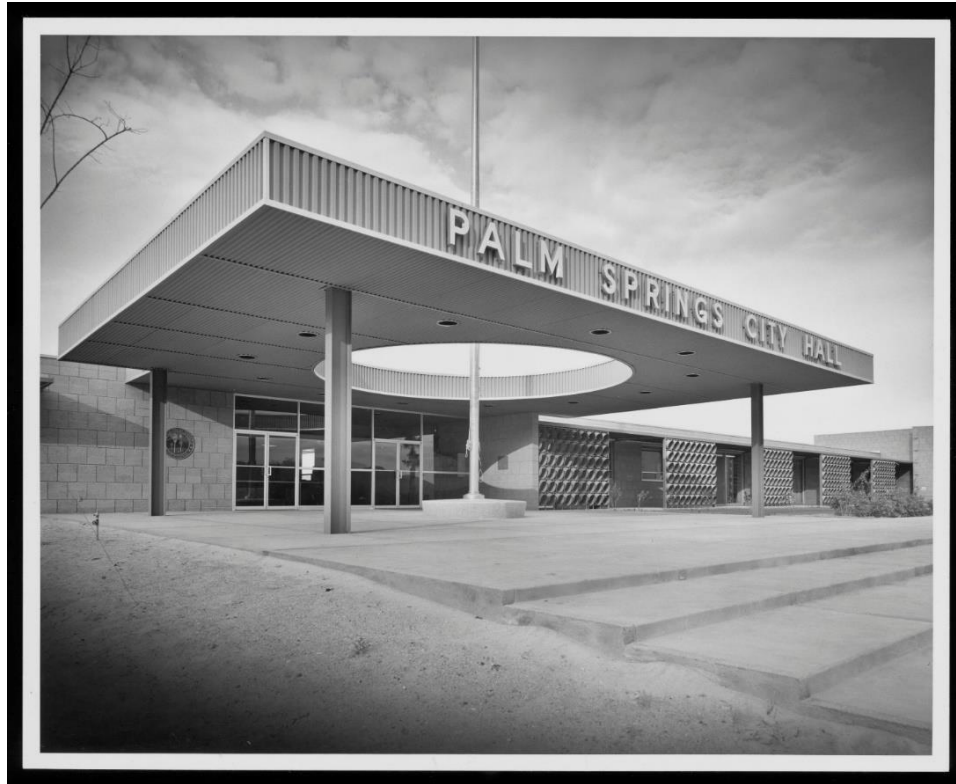
View of front entrance to City Hall, showing flagpole which originally projected through the oculus. The sandy soil of the landscape in front of the Primary Façade – West can be seen directly adjacent to the steps.
