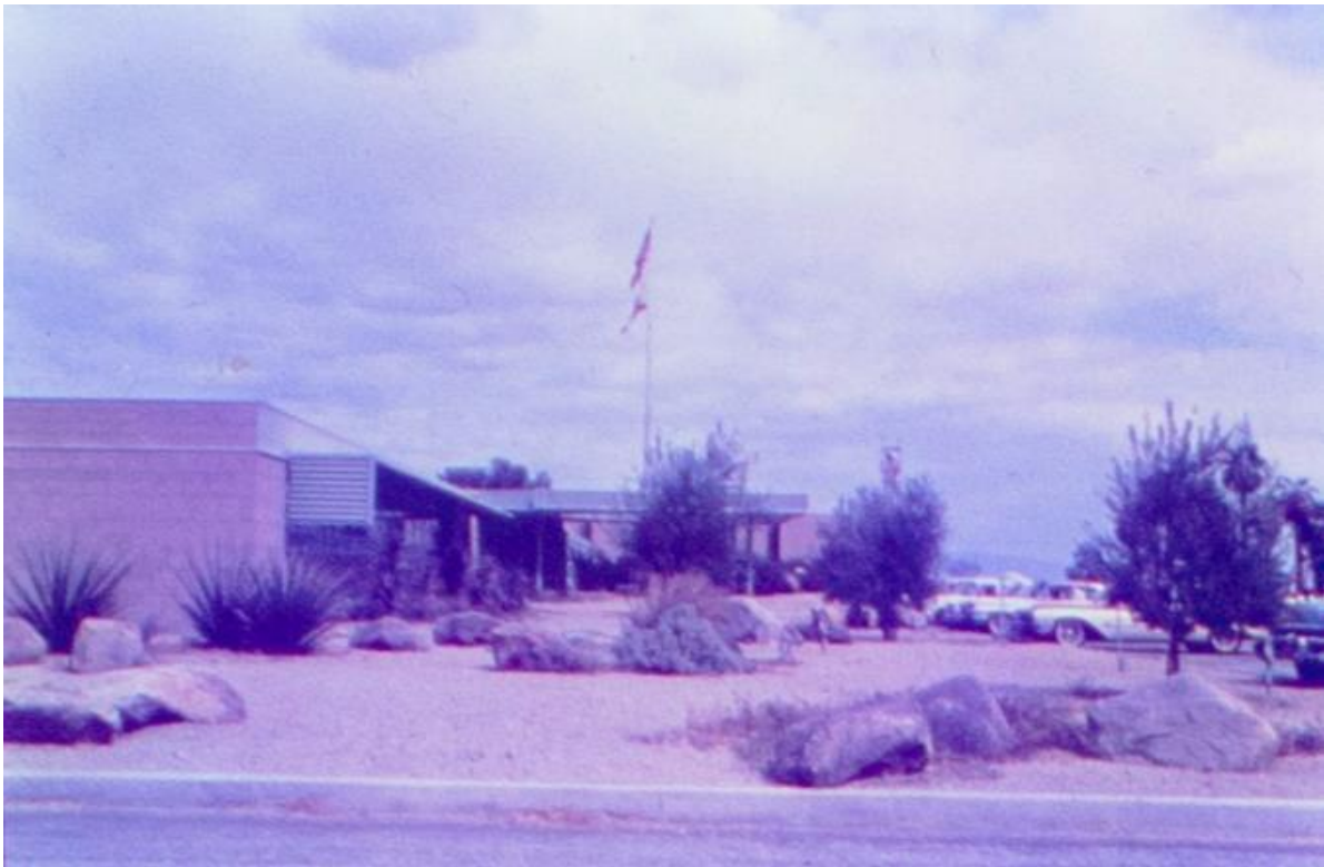
The drought-tolerant landscape at the Primary Façade – West.
