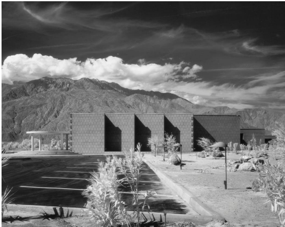
View of the East Parking Lot, facing west.
