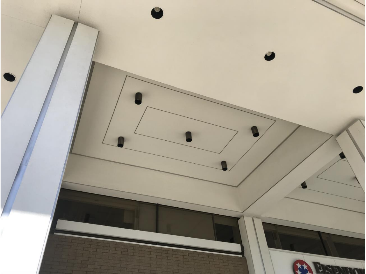
The ceiling of the colonnade has recessed lighting at the perimeter, with five bronze aluminum downlights between each column. Incised lines add decorative detail. Photograph by the author, June 2022.
