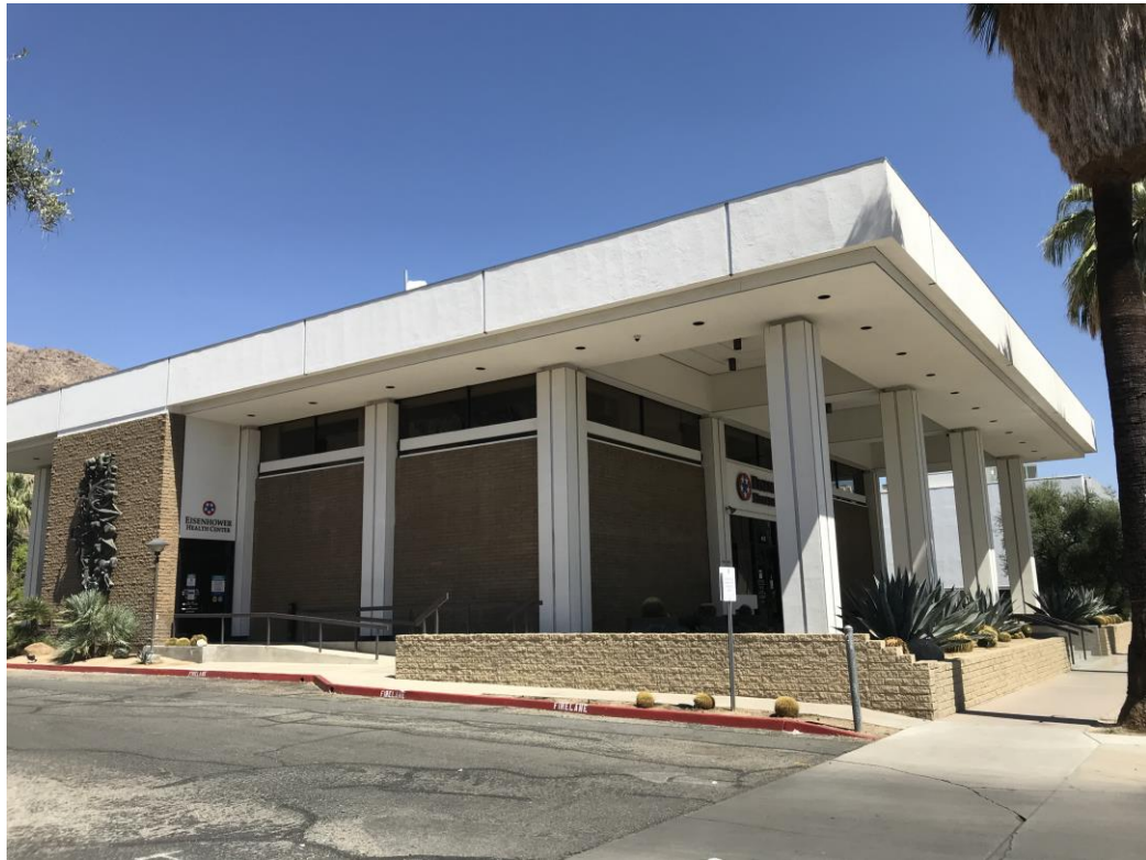
The south façade, showing the tan split-face brick podium, the same brick on the walls, the embedded columns that encircle the structure, the columns supporting the colonnade. Note Abbott Pattison wall sculpture. Photograph by the author June 2022.
