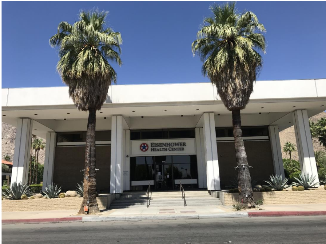
The east elevation of the Merrill Lynch Building faces Palm Canyon Drive. Photograph by the author, June 2022.
