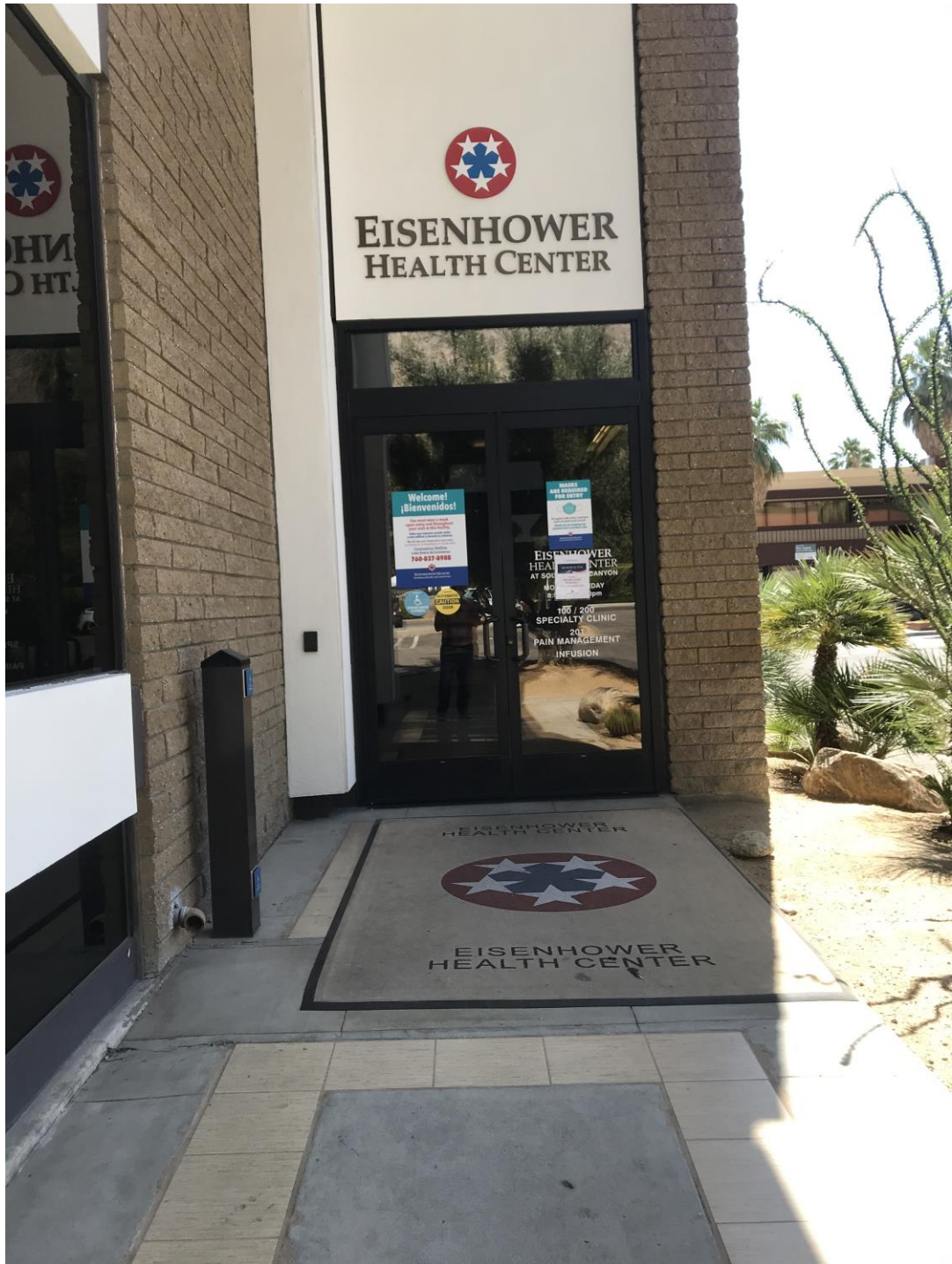
This portion of the building bumps out to the south of the main structure and has entry doors on the east and west sides. Note the tan glazed tiles embedded in the concrete. Photograph by the author June 2022.
