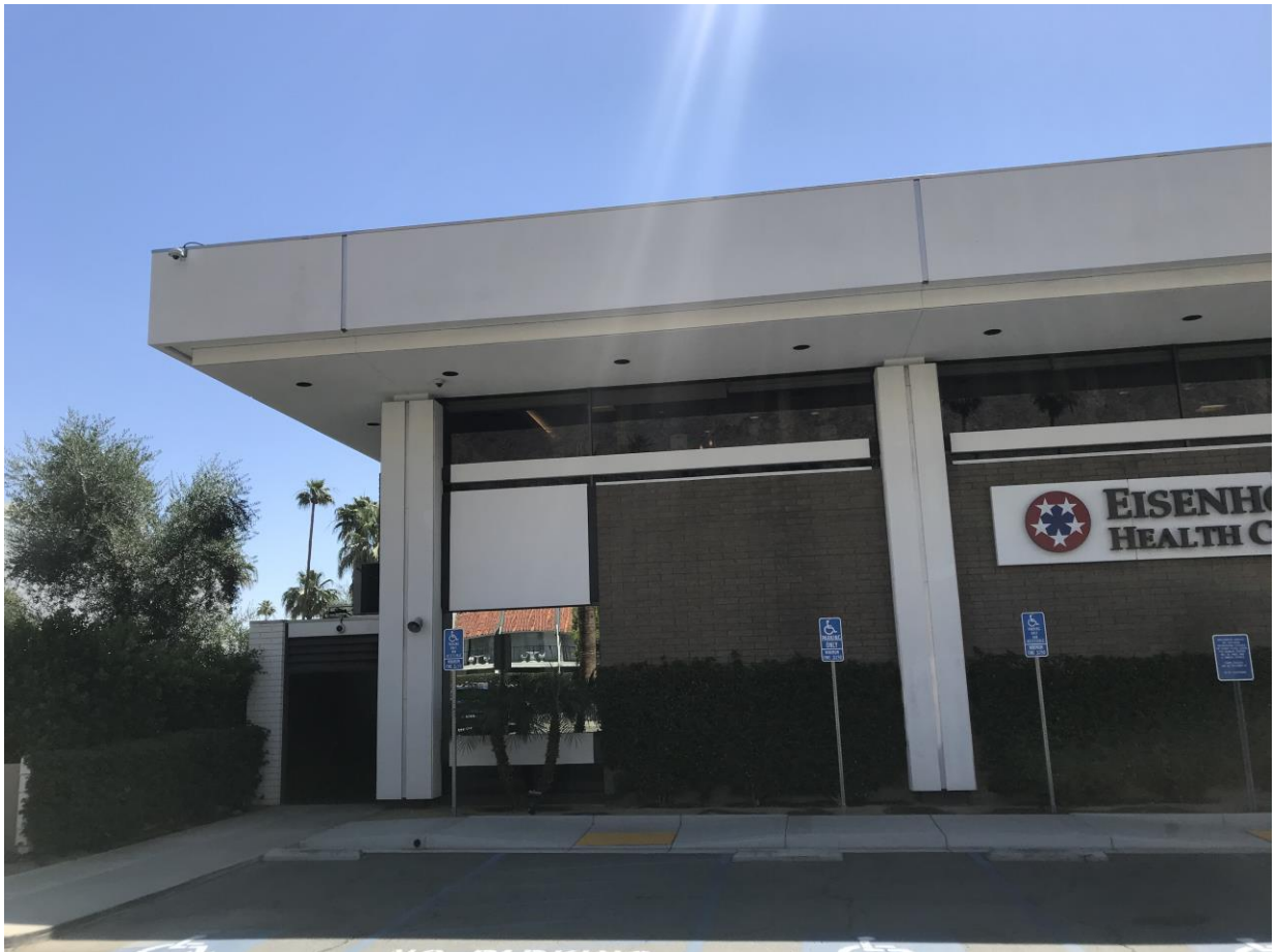
The rear (west) façade with embedded columns supporting entablature (fascia), with walls of tan block, off-white-painted plaster band with bronze-tinted solar glass clerestories. Photograph by the author, June 2022.
