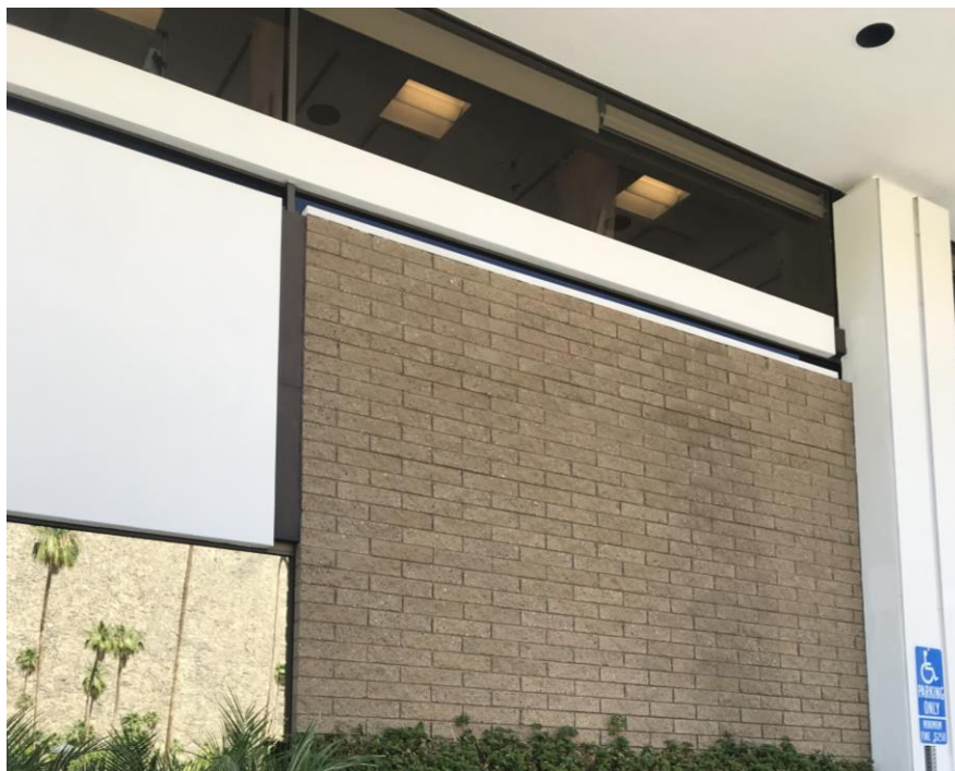
Tan split-face brick, off-white-painted plaster, brushed aluminum, and bronze-tinted solar glass were the materials chosen by Wexler for the Merrill Lynch Building. Photograph by the author June 2022.
