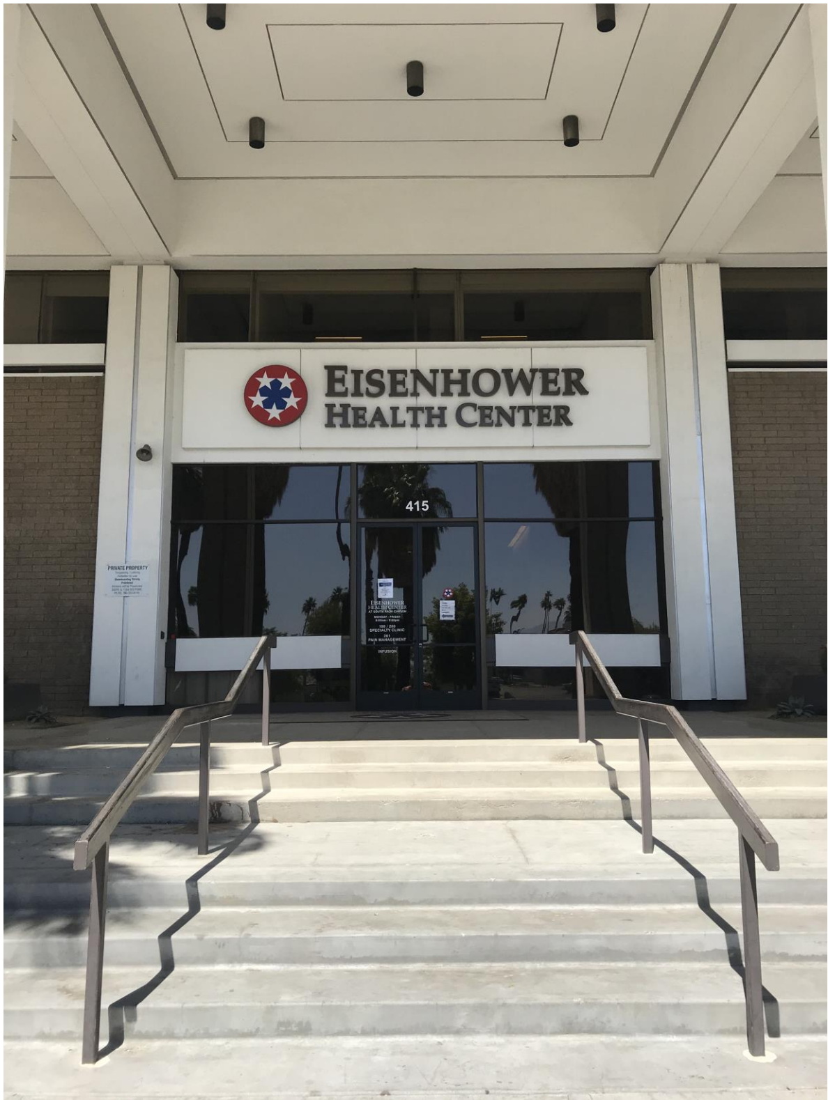
Concrete steps lead up the podium from Palm Canyon Drive to the colonnade. Note the original downlights, a Wexler signature. Photograph by the author, June 2022.
