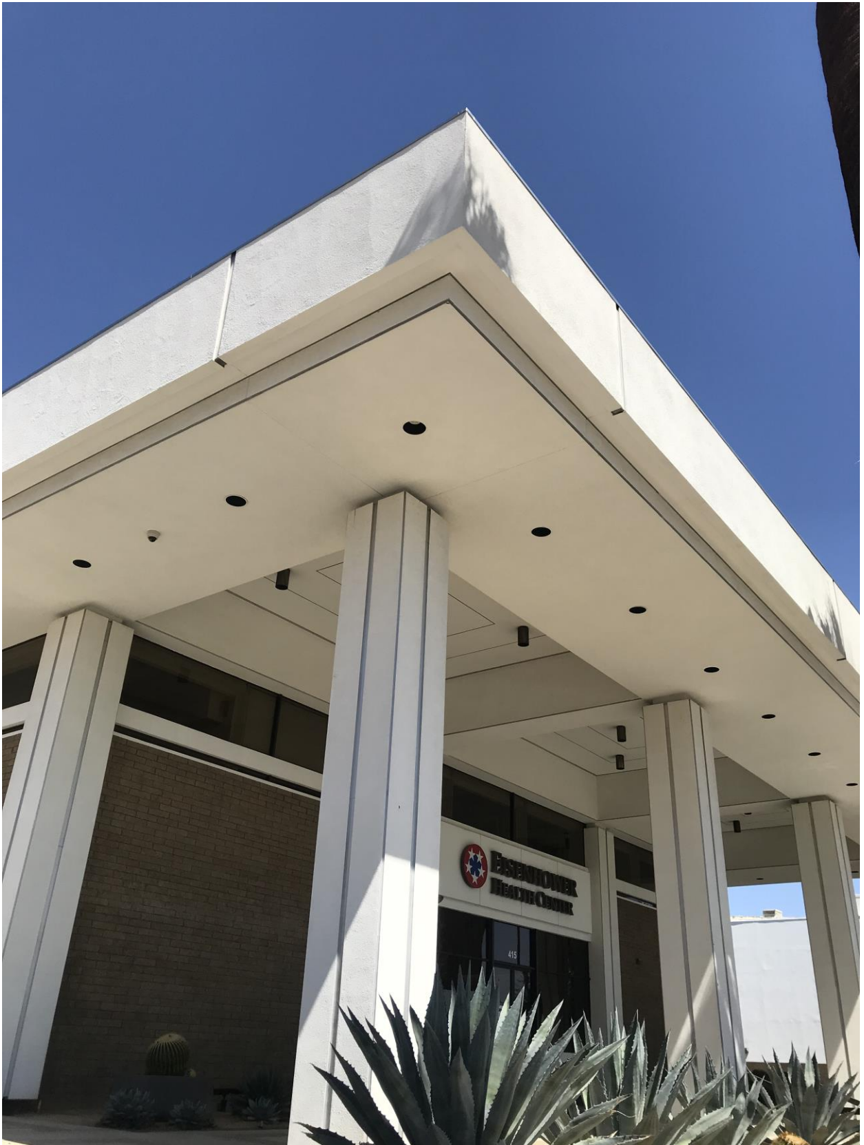
Squared columns with brushed aluminum “U”-channel trim, with matching trim on the fascia. The original juniper has been replaced with a spiky row of yucca plants. Photograph by author June 2022.
