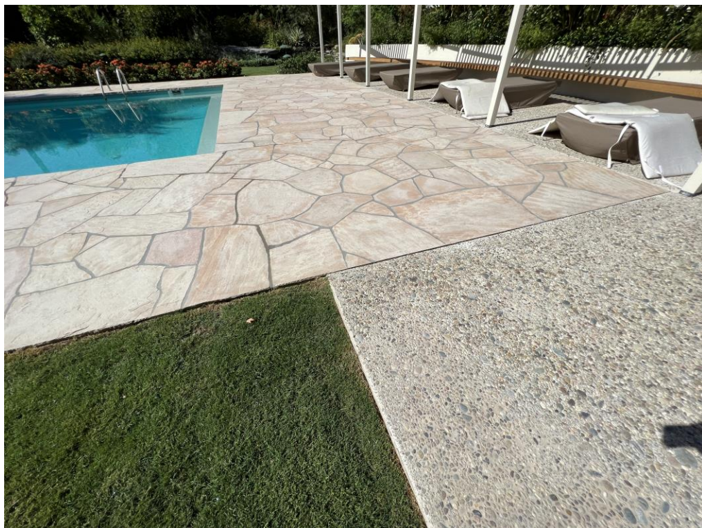
White concrete exposed aggregate contrasts with Arizona sandstone flagstones and a smooth panel of turf.
