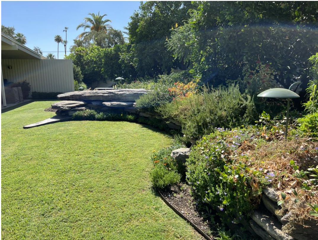
The retaining wall on the south of the property is built using long native stone ledges, naturally varnished a deep coppery brown. Some stones cantilever out, others are embedded in the lawn.
