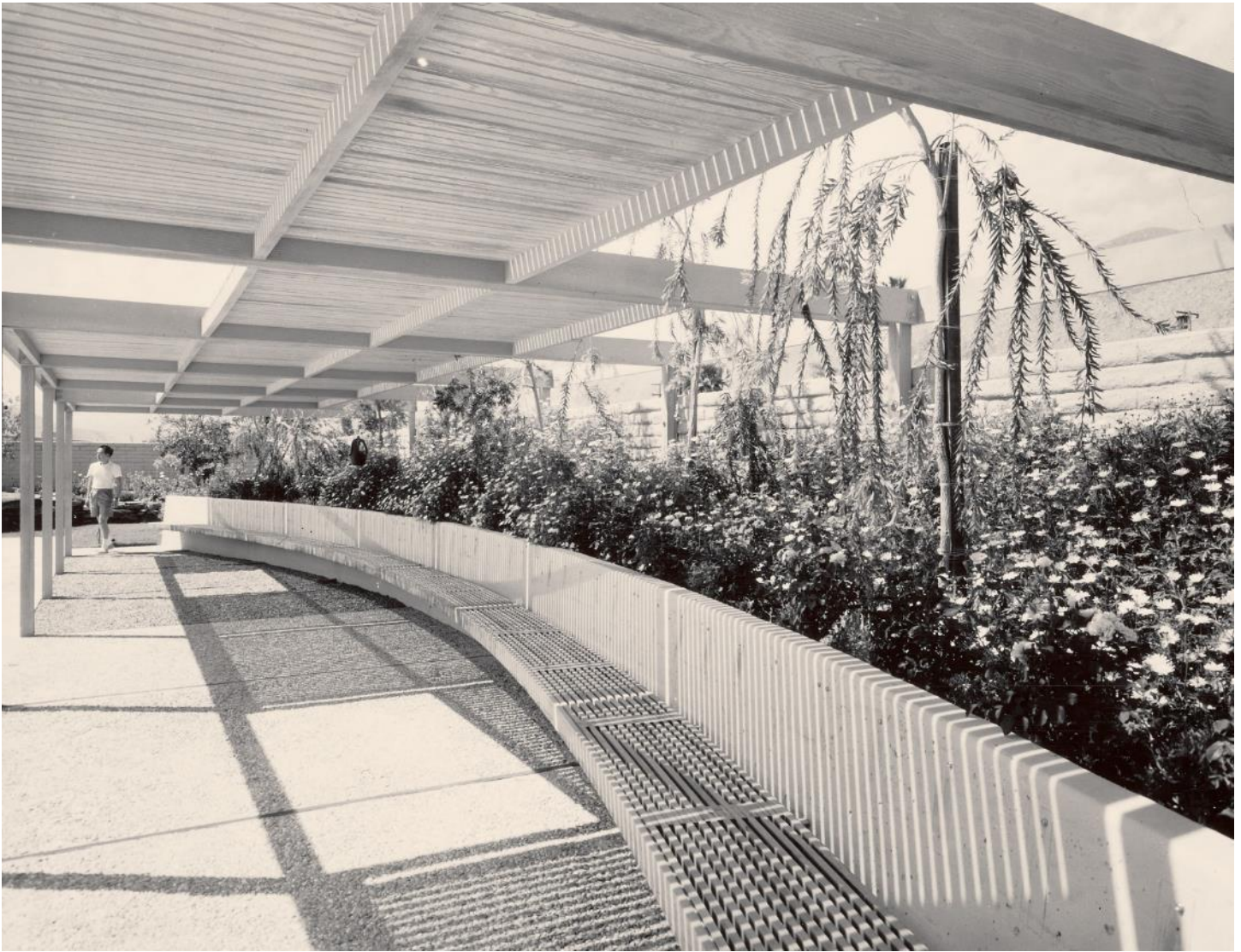
The long slatted wood bench and shade structure. During the recent restoration, this bench and shade structure were completely rebuilt and replicated, using the original drawings as a guide, as well as remnants of the original. Julius Shulman photograph, © J. Paul Getty Trust. Getty Research Institute, Los Angeles (2004.R.10).
