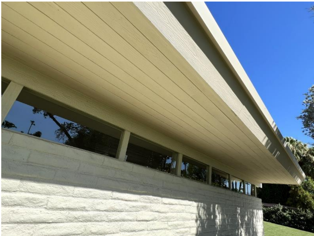
The wood has been sandblasted to emphasize the grain, providing a textural interest.
