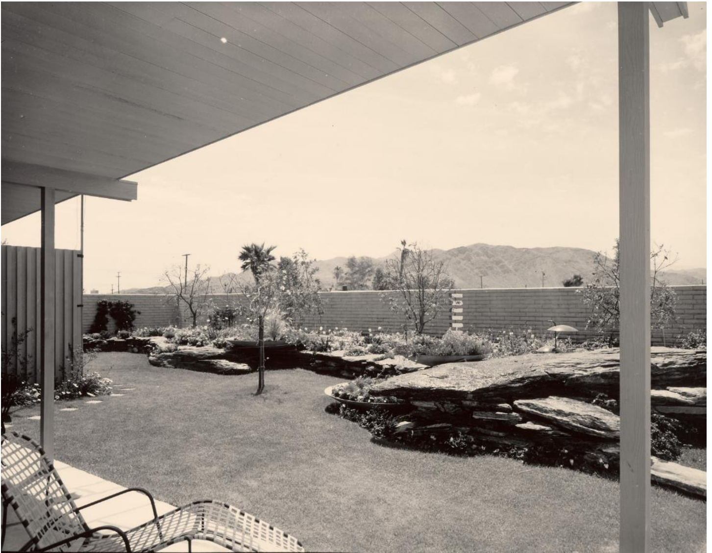
On the south side of the garden, retaining walls were created using varnished native stone slabs. Julius Shulman photograph, © J. Paul Getty Trust. Getty Research Institute, Los Angeles (2004.R.10).
