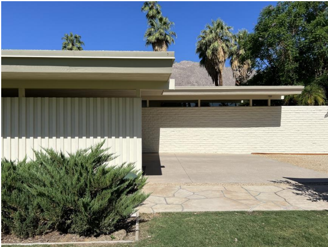
Sandblasted board-and-batten is combined with Slumpstone.
