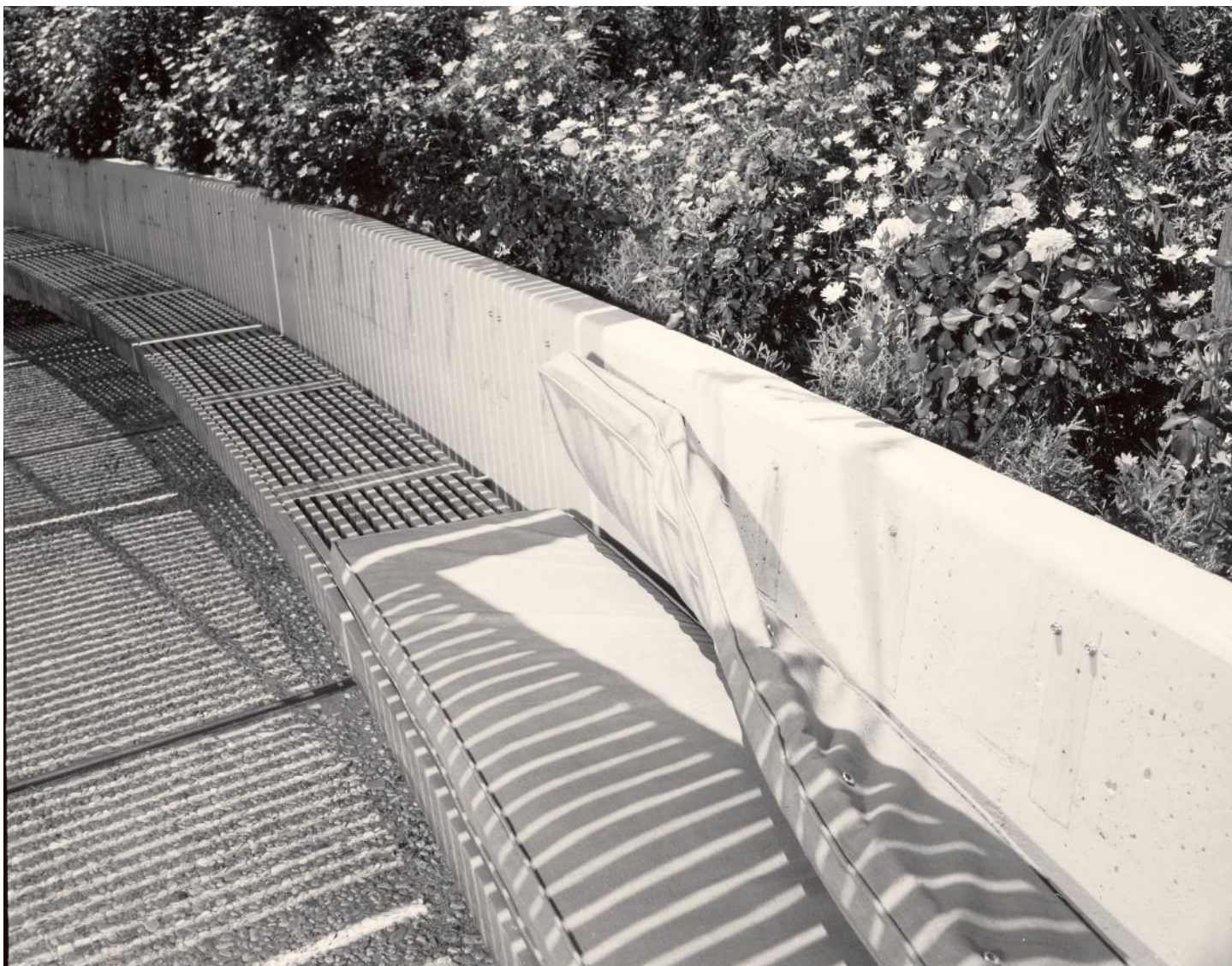
Canvas fabric cushions were attached with special hardware to the poured concrete wall back of the bench. Julius Shulman photograph, © J. Paul Getty Trust. Getty Research Institute, Los Angeles (2004.R.10).
