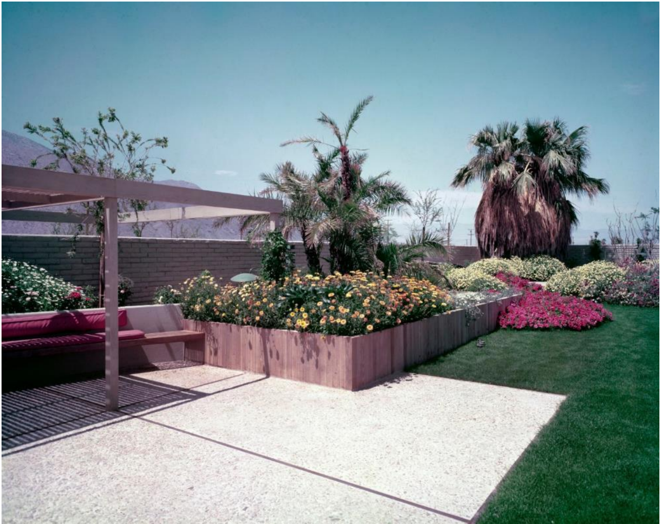
The paving at the shade structure was white concrete exposed aggregate. Redwood planting box, with contoured earthforms in the background. All of the features seen here were meticulously restored. Julius Shulman photograph, © J. Paul Getty Trust. Getty Research Institute, Los Angeles (2004.R.10).
