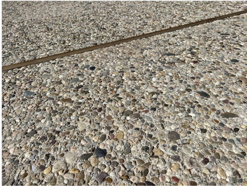
Eckbo and Dean specified white concrete exposed aggregate at the bench and shade structure. This was carefully replicated when the garden was recently restored.
