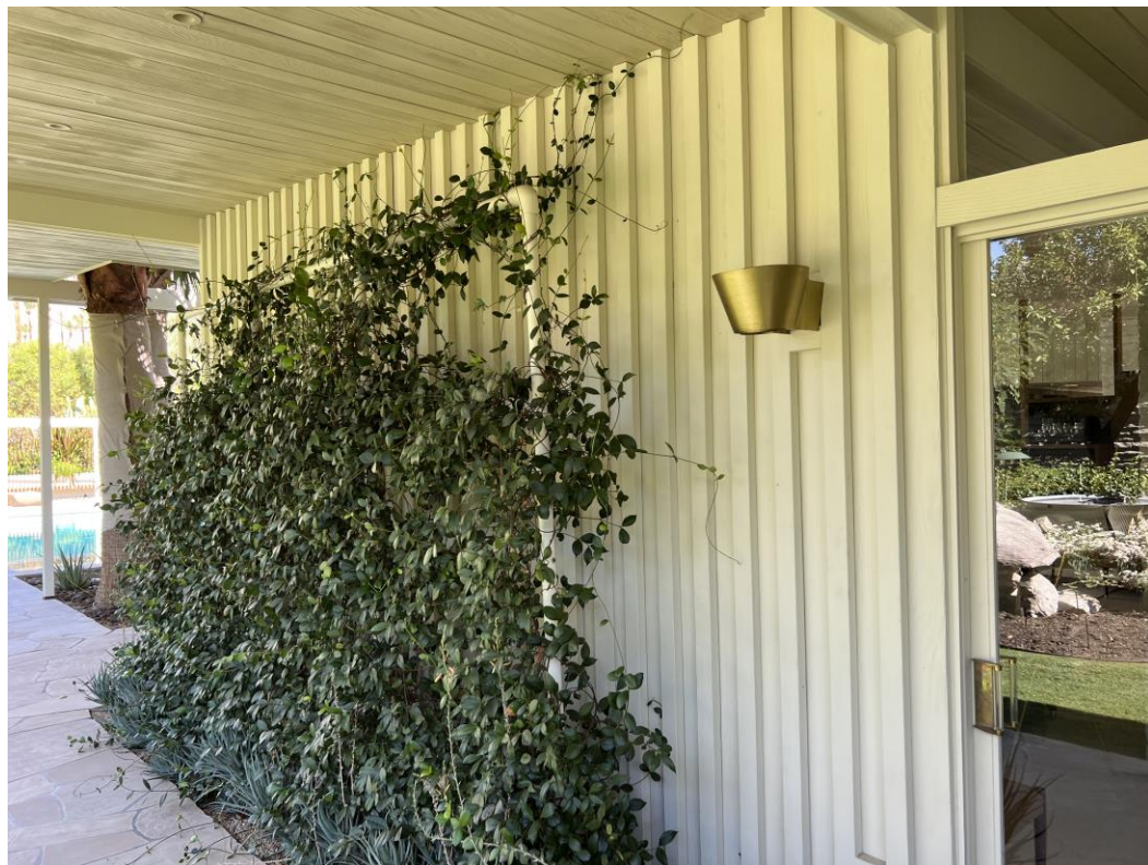
Another Paavo Tynel sconce, and board-and-batten vertical wood detail. Eckbo and Dean created a simple trellis using pipe and wire, trained with jasmine.
