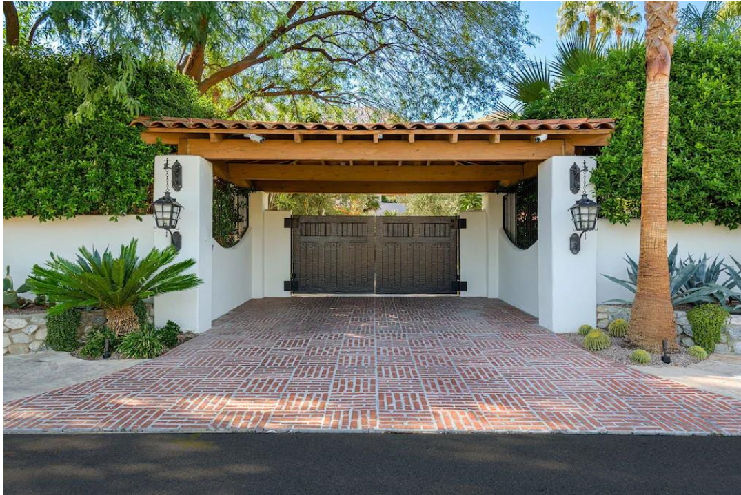
The entry portal to the driveway. This is a non-contributing element created in 2001.
