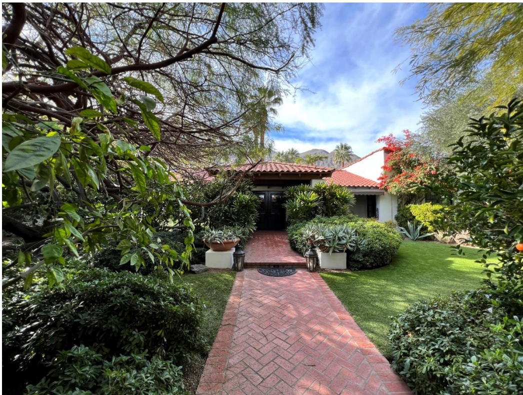
The primary façade today, with shed-roofed dining wing showing through foliage at right; original covered front porch; and the later entry addition at center.
