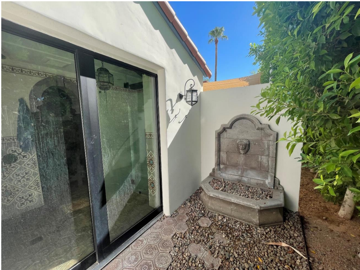
Sliding glass door and private patio with fountain outside the Hicks' 1971 primary bedroom addition.
