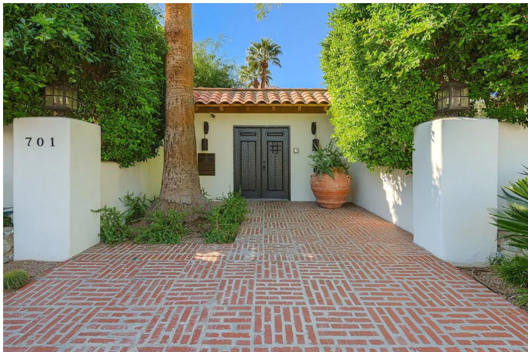
The entry portal to the front door of the home. This is a non-contributing element created in 2001.
