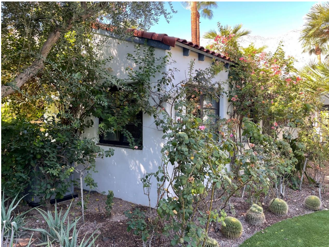
The northeast corner of the 1926 portion of the house. Off-white painted stucco walls, wood casement windows, and thin roof elevation covered in red tiles.
