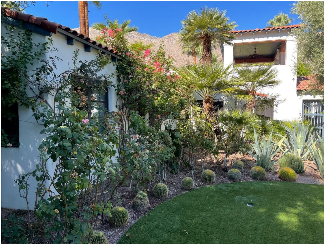
The original 1926 north elevation, faces the driveway, with the 1936 tower beyond.
