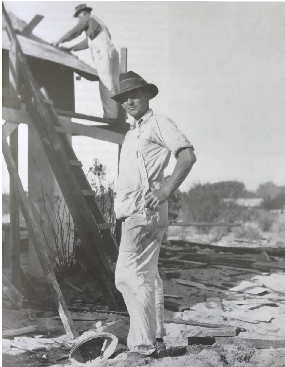
Alvah Hicks photograph during construction of the Kellogg Residence. Courtesy Palm Springs Historical Society.
