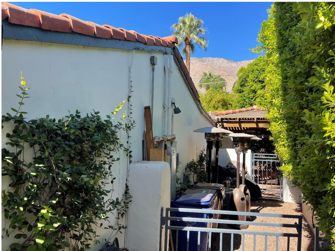
The north façade of the 1926 garage structure.
