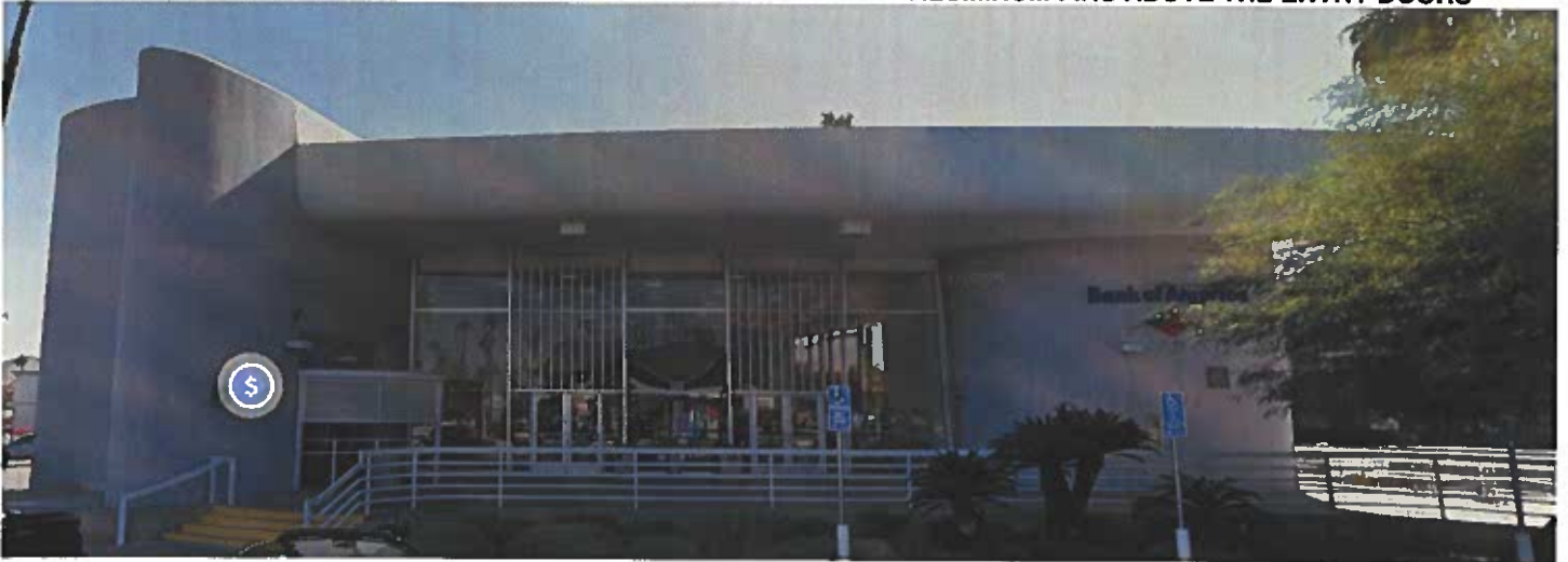
BELOW: THE NORTH ELEVATION OF THE BANK SHOWING THE ALUMINUM FINNS ABOVE THE ENTRY DOORS
