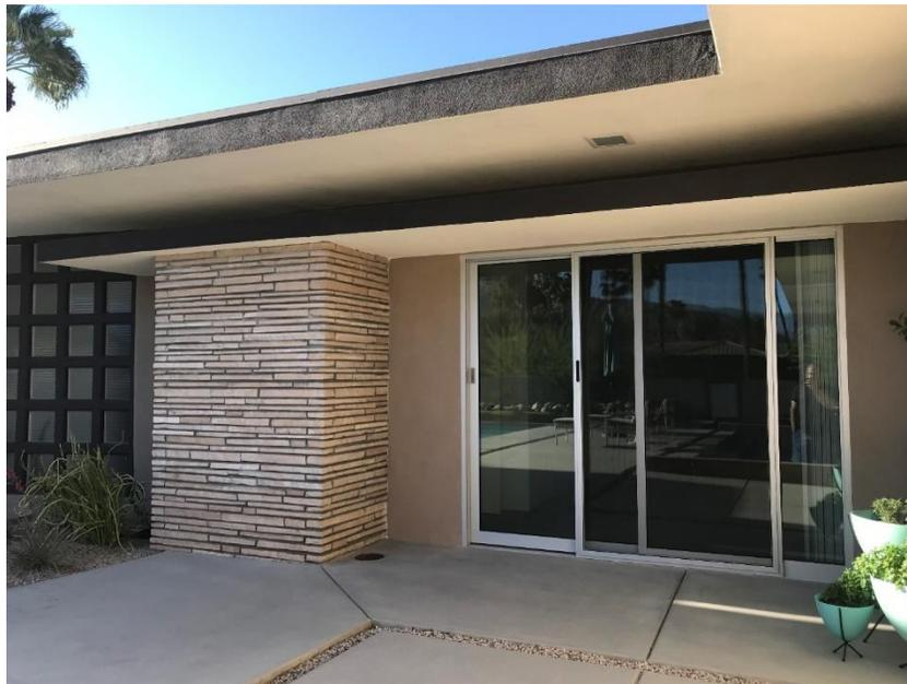
*Top: In this February 2019 photo, the secondary roofline had been recently demolished. This was originally supported by one of Herbert Burns' distinctive Arizona sandstone piers, but that feature had been removed in the past and turned into a doorway.*
