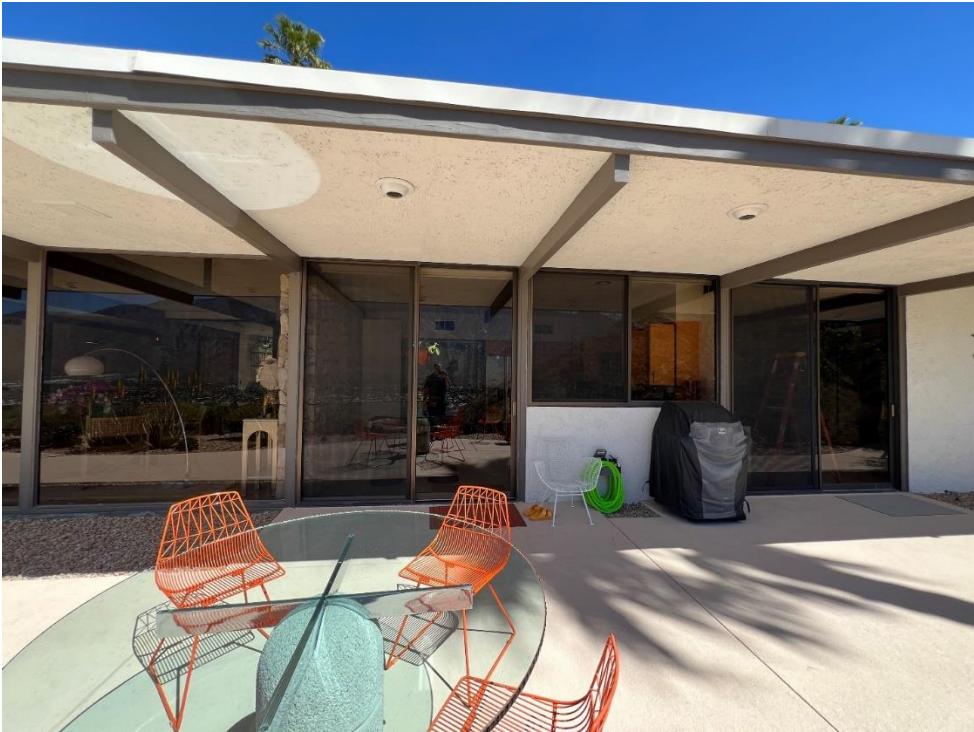
Exterior wall showing kitchen area.
