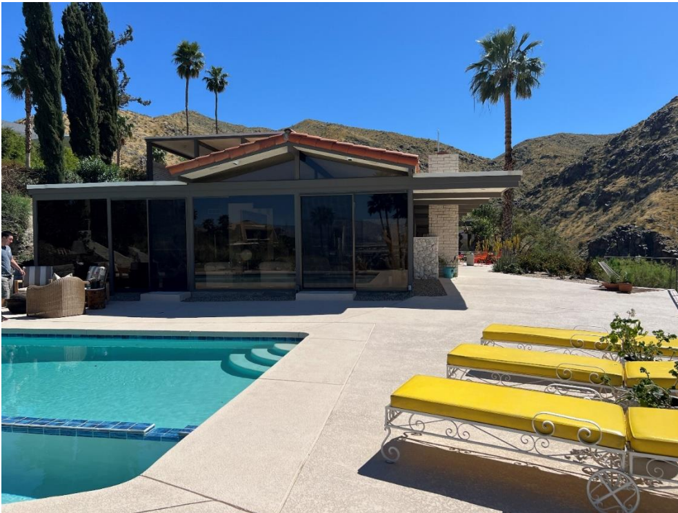
South facing façade shows post-and-beam house with pitched roof volume.
