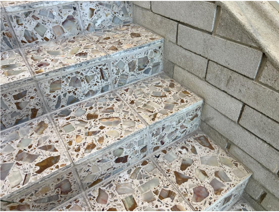
Detail of the entry stair terrazzo tiles.
