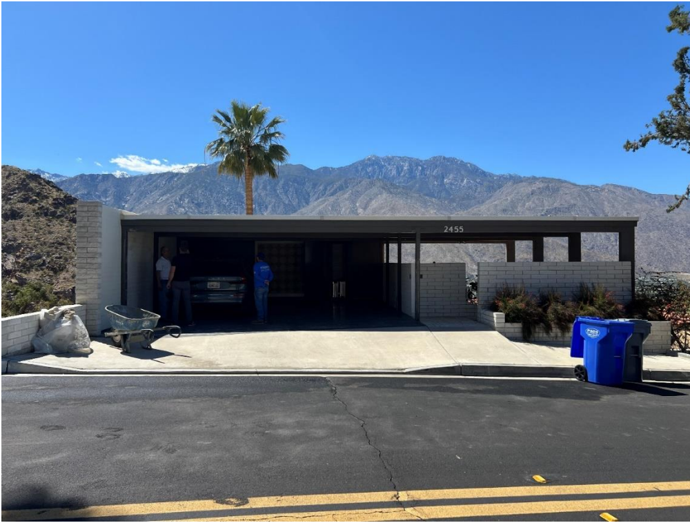
Looking west from Southridge Drive, showing carport and entry stairs.
