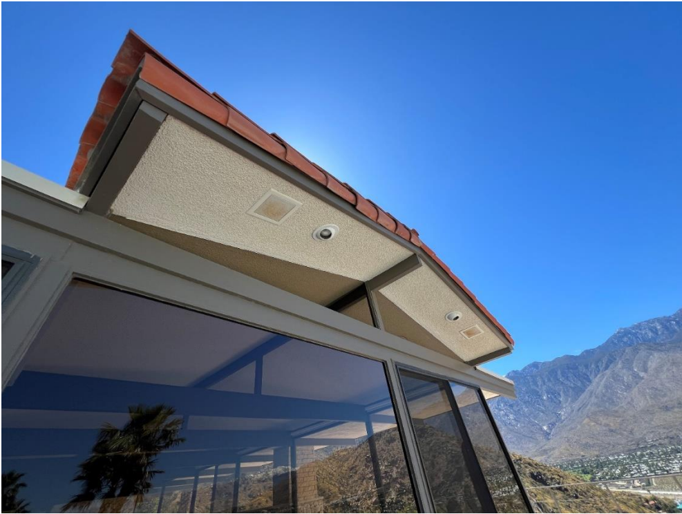
Pitched clay tile-roofed volume of living room, with bronze-anodized sliding glass doors.
