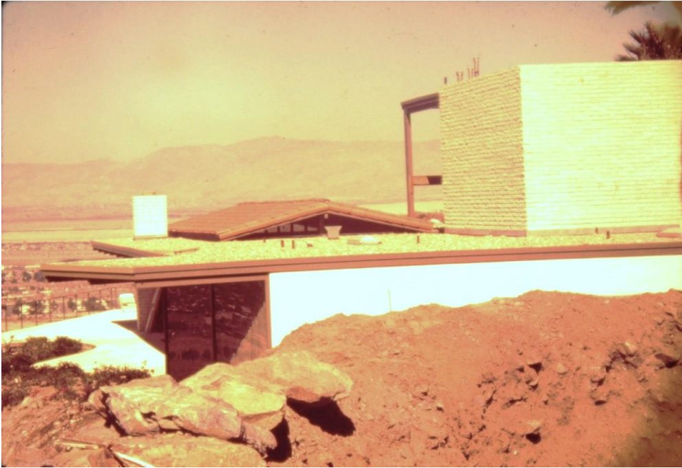
November 1971 – House during construction
