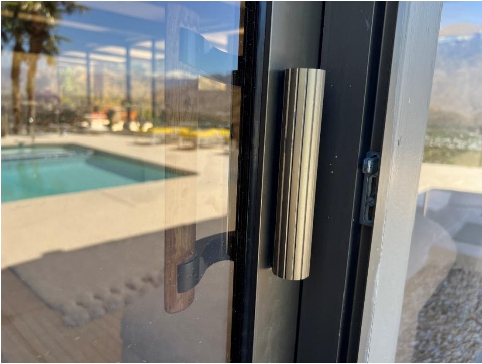
Door hardware detail, bronze-anodized sliding glass door.
