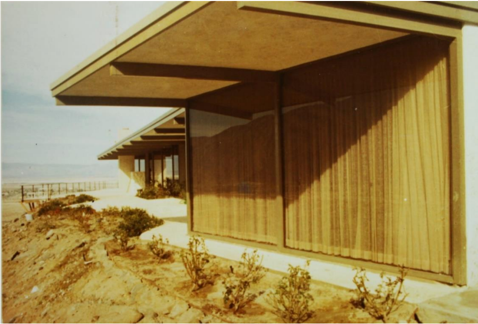
1972 – Newly completed house showing bedroom windows and western façade.
