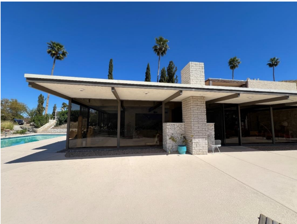
West façade showing Dolomite stone veneer on fireplace, with chimney constructed using the same off-white split-face block as the house.
