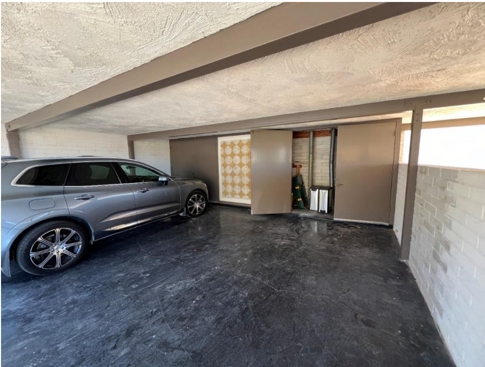
Post-and-beam carport with storage closets at rear.
