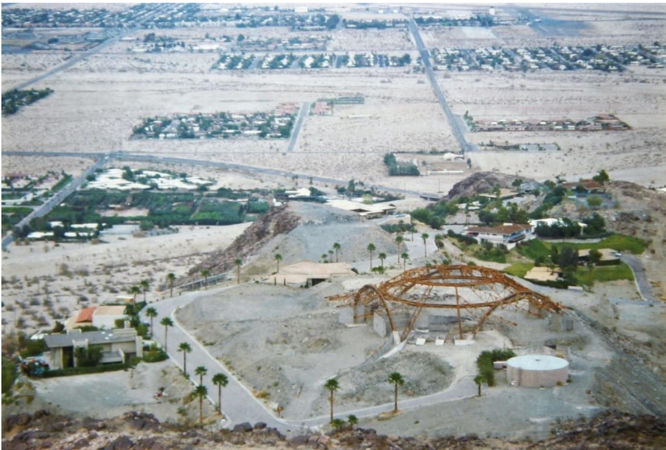
December 1975 – Garber Residence at far left, showing construction of the John Lautner-designed Bob Hope House.
