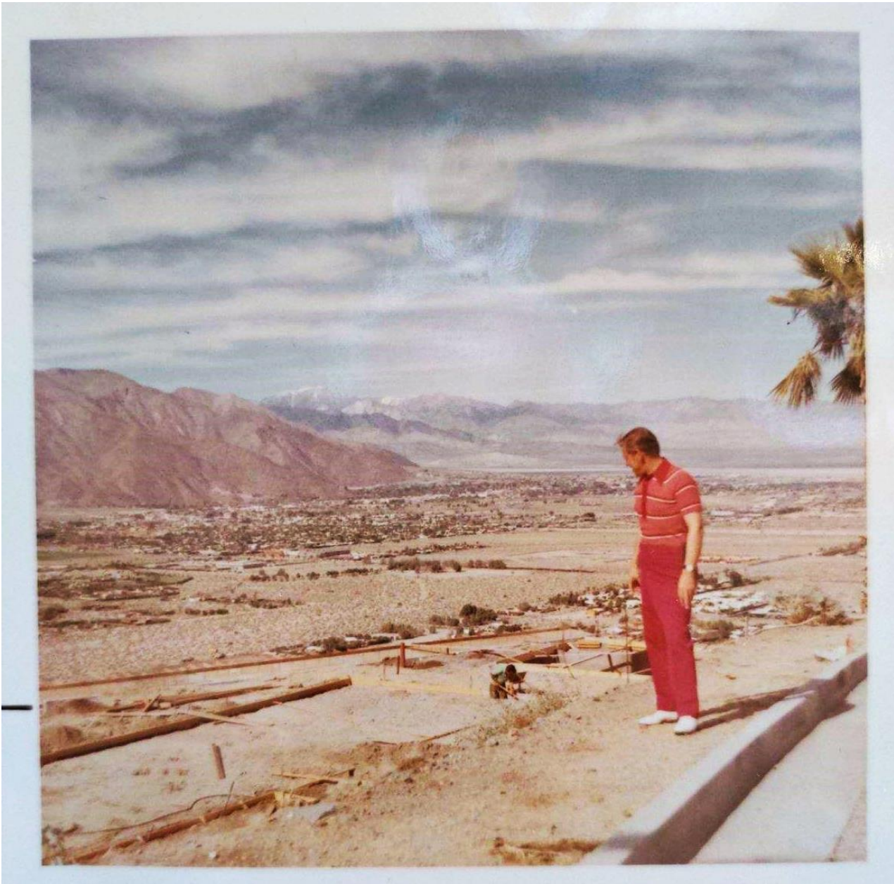
Early 1971 Harry Garber looking at early construction
