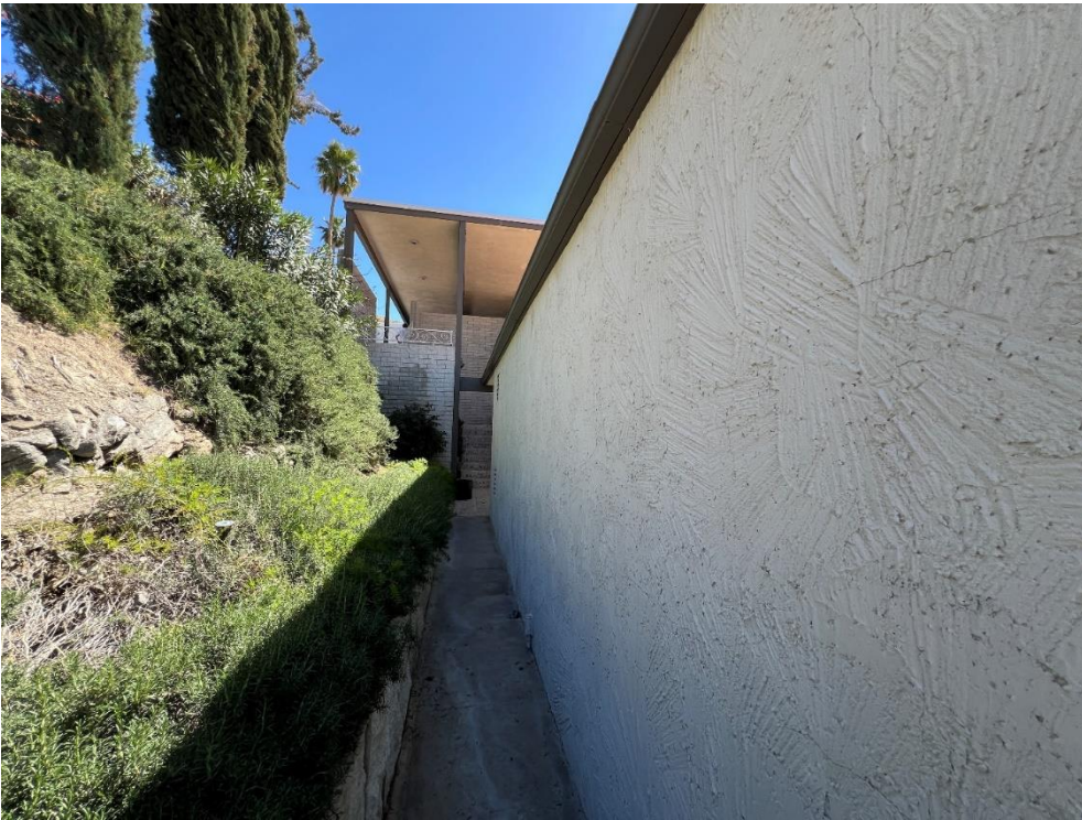
The long corridor leading from entry area toward pool area.
