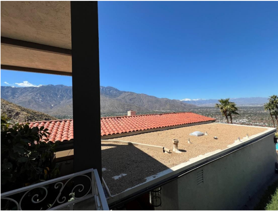
View northwest over the house from the entry stairs.
