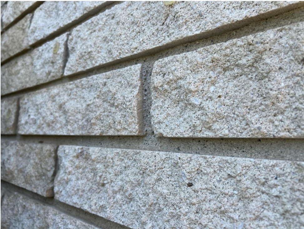
Detail of the off-white split-face concrete block
