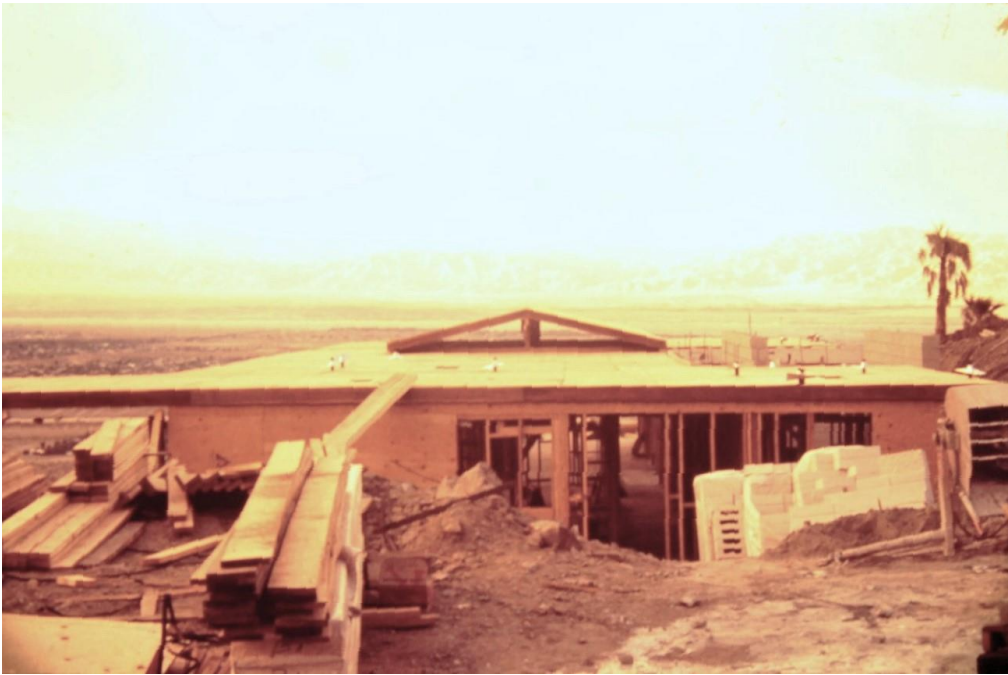
April 1971 – House during construction
