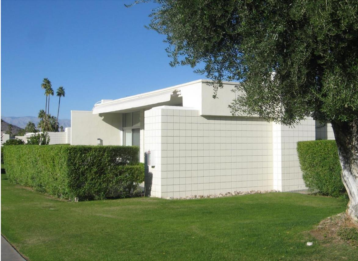
**View showing some of the ways in which Jones mixed concrete blocks with smooth masonry. Note the difference in patio wing walls and overhanging roof, which cleverly hid air-conditioning systems.
