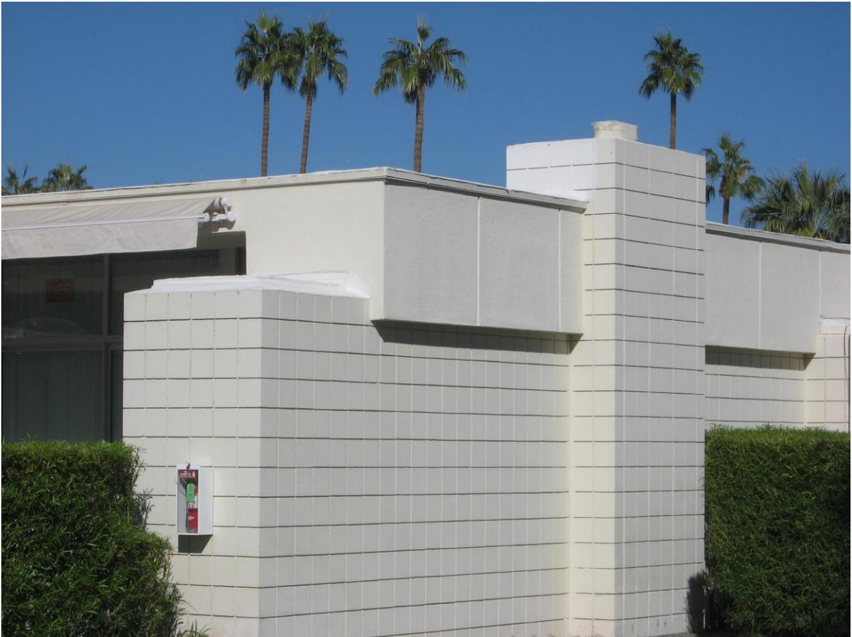
**A section showing a portion of roof scored to mimic concrete blocks below. Note how the architect enlivens the massing in the way the roof is pulled out from the façade. Fireplace also adds to this effect.**
