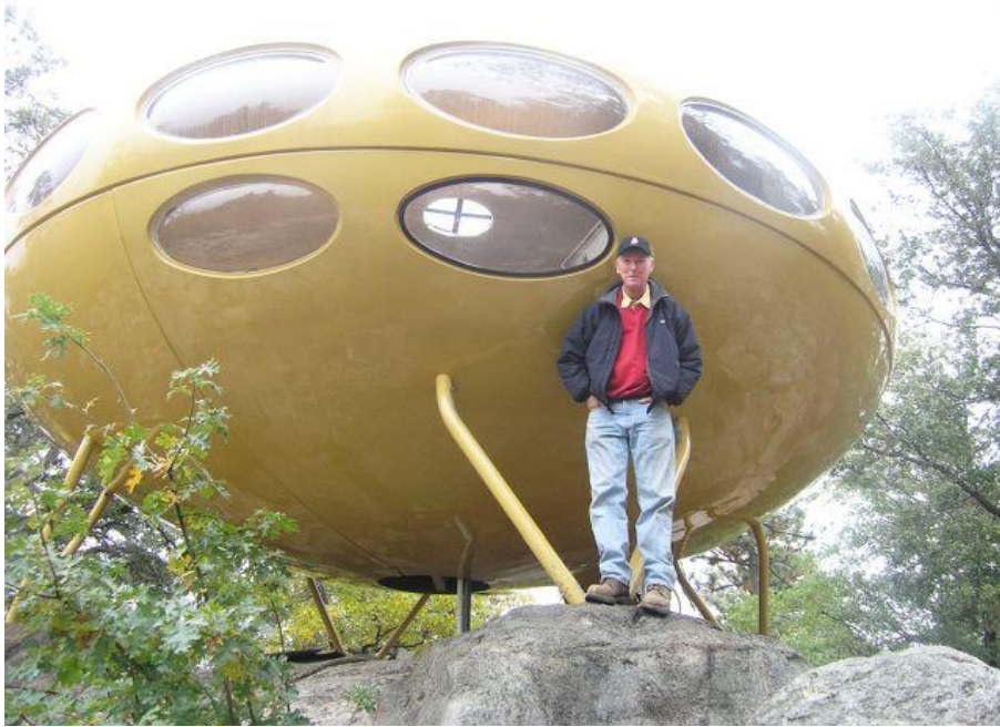
Wayne Donaldson has worked for many years to get his award-winning restoration of the Futuro accomplished. Here he is seen in 2006 with the futuristic home. Photo by Dave Weinstein.
