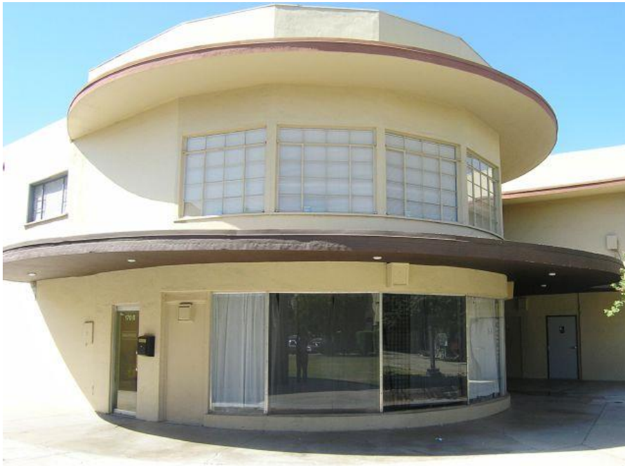
The Palm Springs Preservation Foundation has been working for decades to save the Town and Country Center, which was designed by A. Quincy Jones and Paul R. Williams, from demolition and death by neglect. This curve is characteristic of Williams' designs. Photo by Dave Weinstein.
