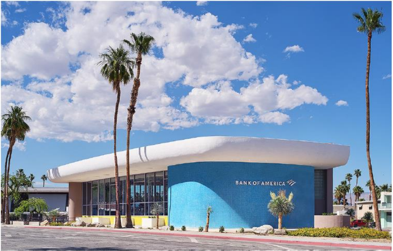
Newly restored Bank of America Palm Springs Main at 588 S. Palm Canyon Drive in 2024
