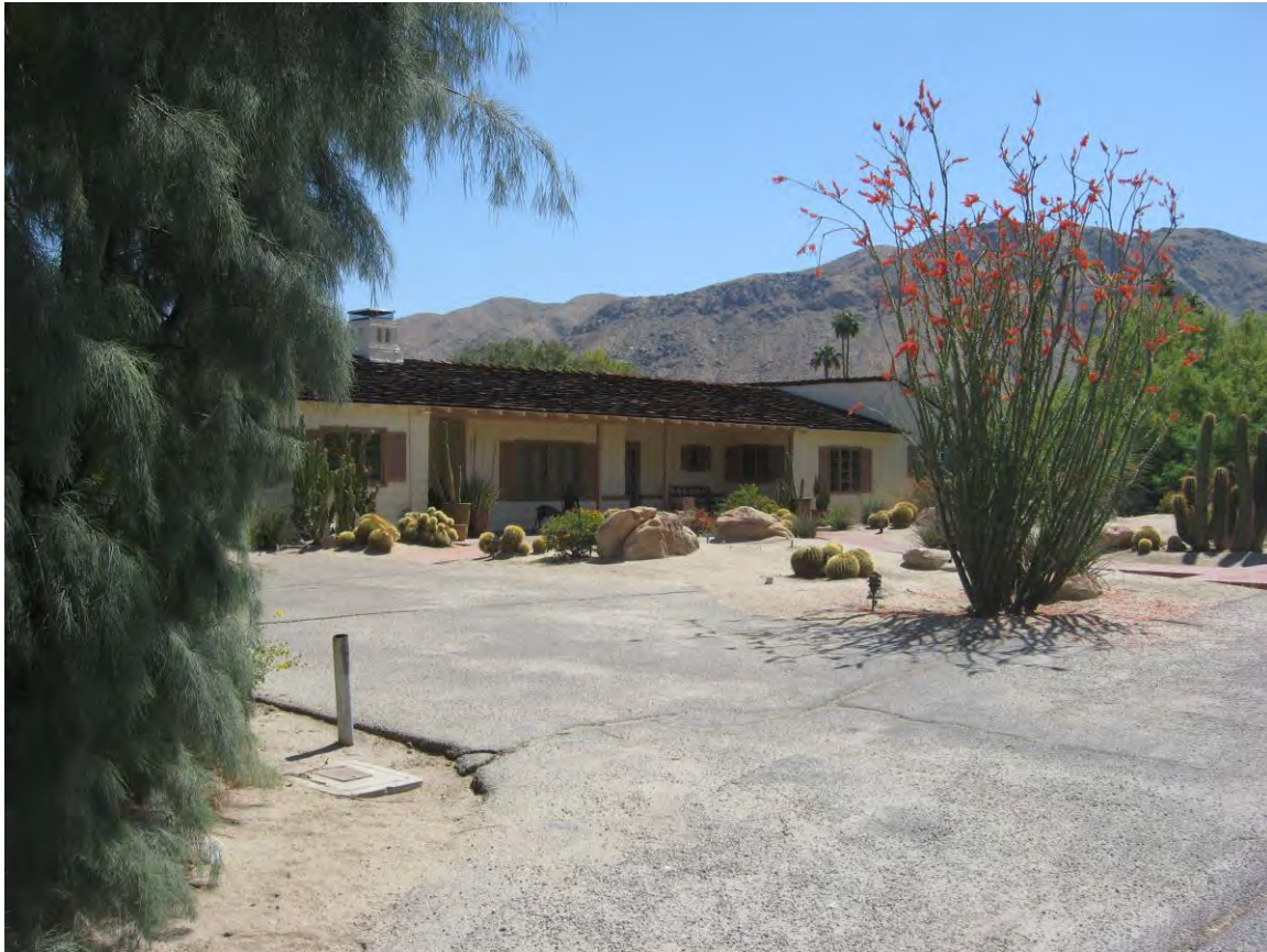
View looking towards west (front) façade. Note the shed roof, deep porch and original fireplace chimney. (Author photo. April 2022)
