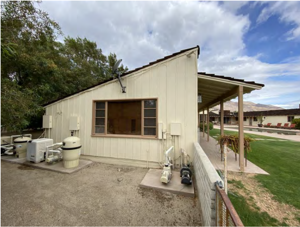
Photo 11. View of 1956 studio addition looking west. Note shed roof designed to match original 1930 design. (Thomas Morbitzer Photo. April 2021)
