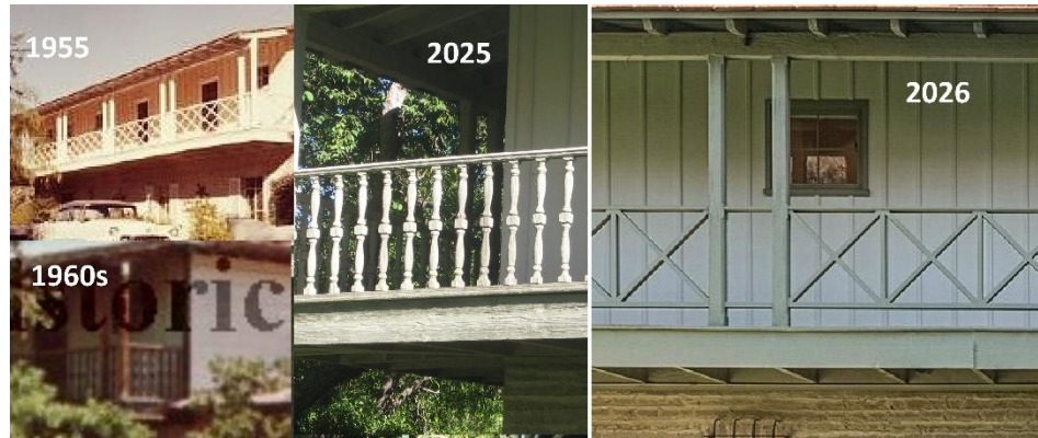
These images show how the balusters have changed from 1955 to the present.
