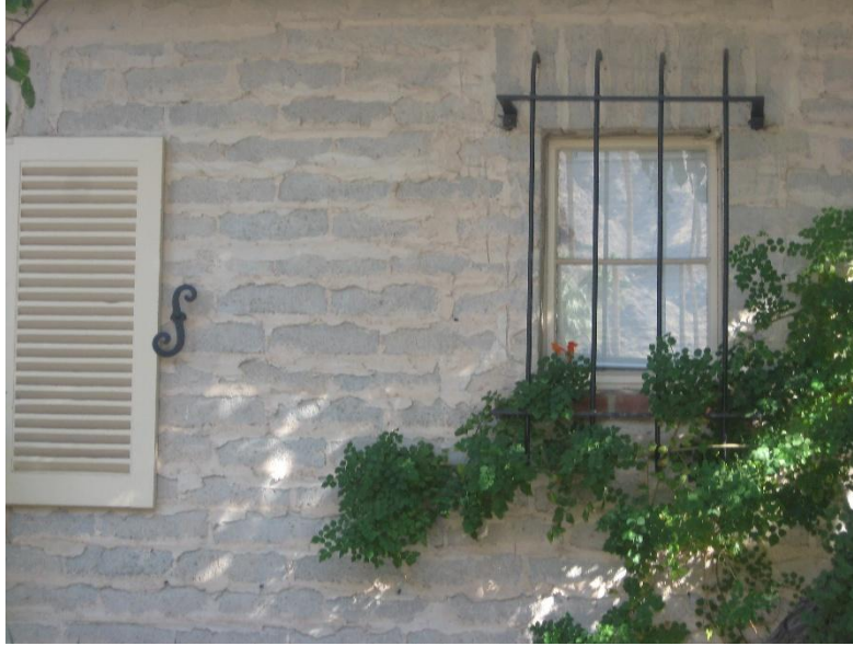
Detail of brickwork on the façade showing the rusticated manner of the troweling between courses. Note how Matcham used red brick as a contrast for the window apron and the use of wrought ironwork. (Author photo. August 2025)
