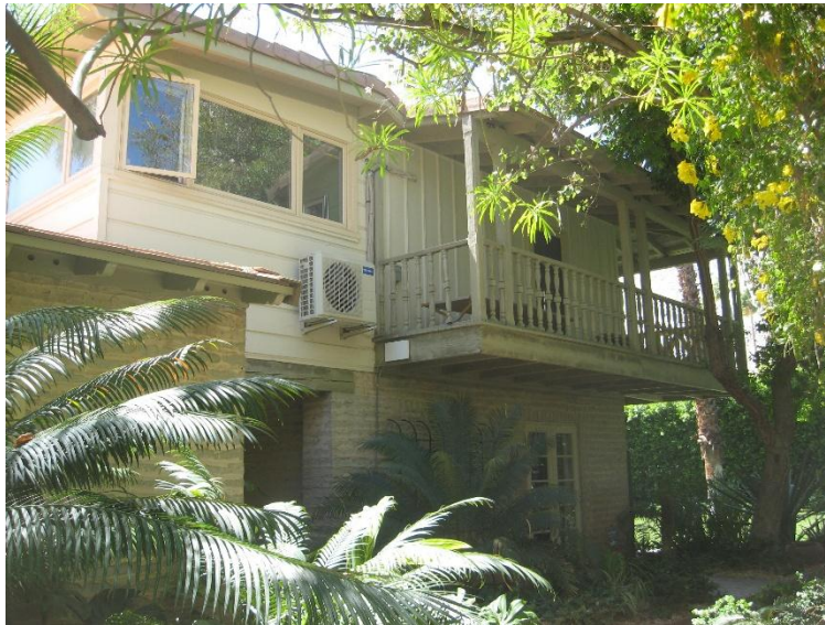
The home's northern façade shows how Matcham switched the orientation of the board cladding from vertical to horizontal. (Author photo. August 2025)
