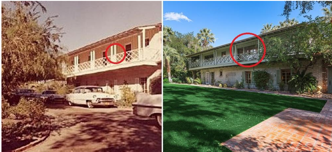
Comparisons between the image on the left dated June 1955 and 2026, on the right, show a set of windows added between the doors (above the rocking chairs).
