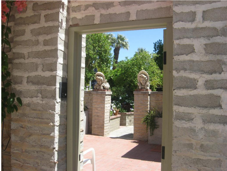
A view looking into the enclosed patio between the main house and garage shows different wall types. Note the foreground wall shows evidence of having been raised higher at some point. Below image shows brick wall separating motor court and front grounds (Author photos. August 2025)
