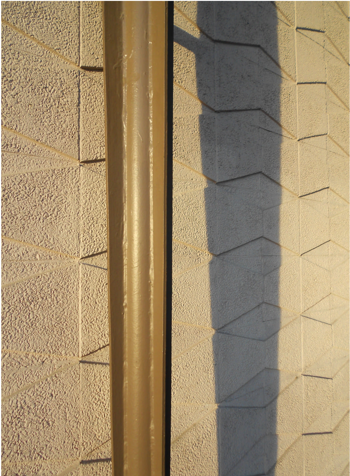
Figure 9: Load-bearing 4-inch “finned” steel pipe columns and harlequin-patterned facing tiles (2012)
