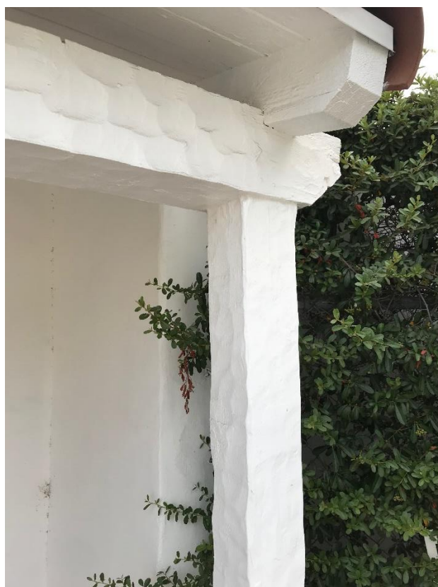
The rusticated posts and beam on the front of the Gate Lodge.
