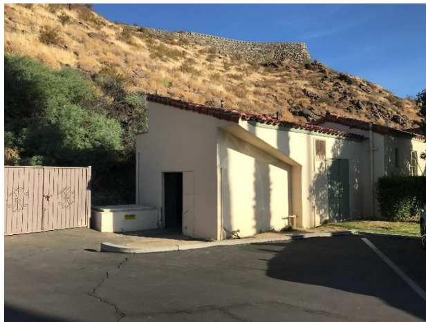
When the south wing was demolished, this shed-roofed structure was cut off and new wall with door added.
