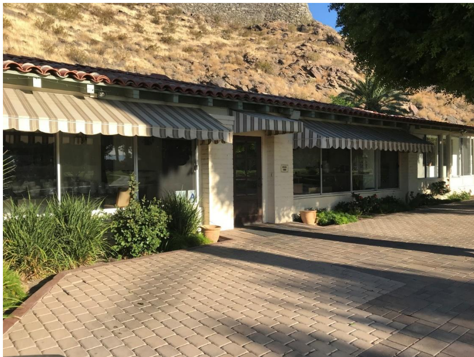
Heavy masonry pilasters paired at entrance, with a single pilaster to the north. Pairs of vertical wood supports line the arcade at the remainder.
