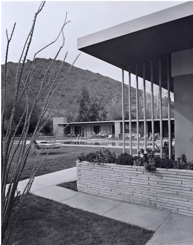
Herbert Burns' Late Moderne detailing at the Town & Desert Apartment Hotel, 1947. PHOTOGRAPH BY JULIUS SHULMAN, © J. PAUL GETTY TRUST. GETTY RESEARCH INSTITUTE, LOS ANGELES (2004.R.10)
