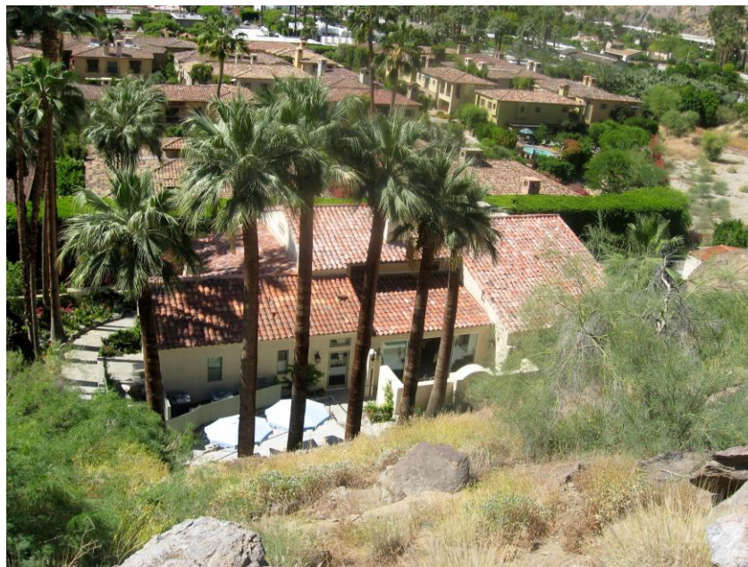
This view looking south shows the multiple intersecting rooflines of the Bishop House. The lowest roof at center covers the dining room.
