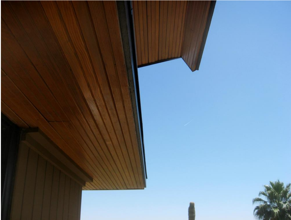
Photo 15: Detail of light shelf and cambered roof above. (Author Photo. May 2020)
