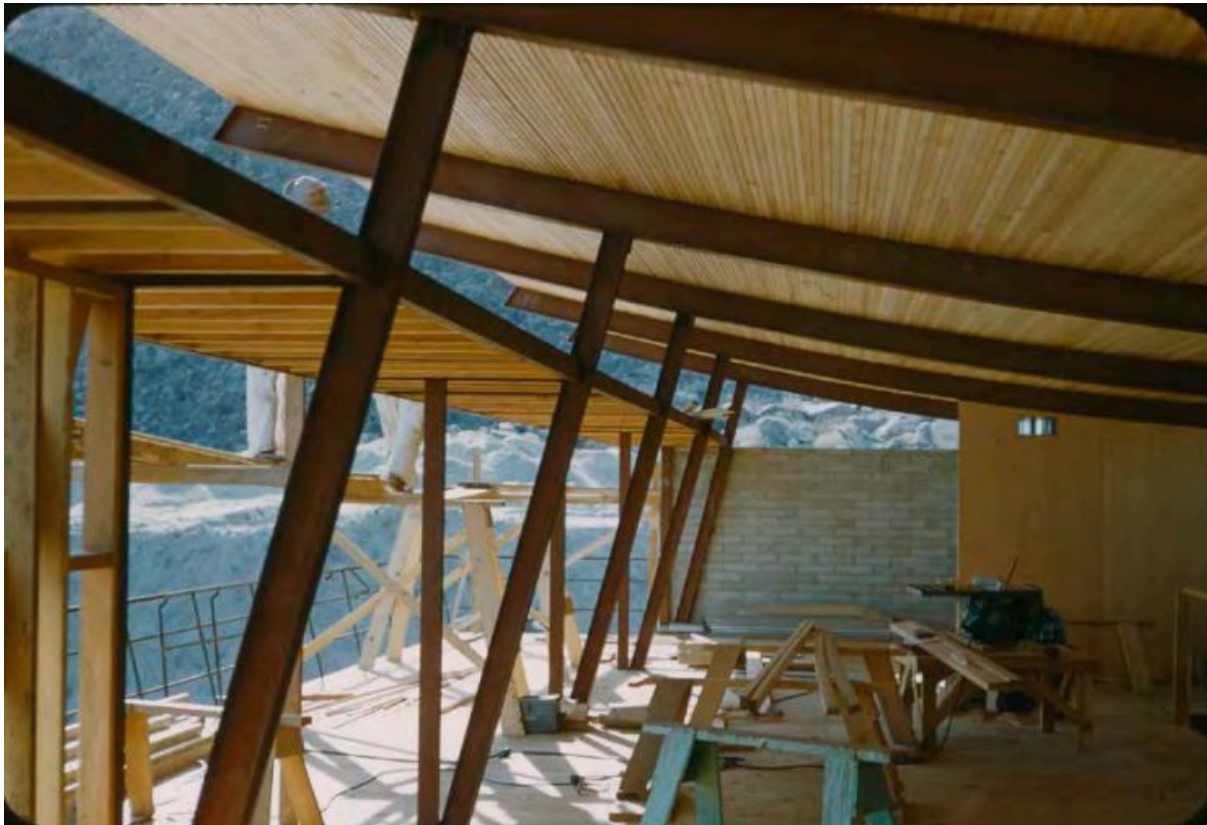
A mid-construction view showing how the steel framing, the light shelf and roof connect. (Walter S. White papers, Architecture and Design Collection; Art, Architecture and Design Museum; University of California, Santa Barbara)
