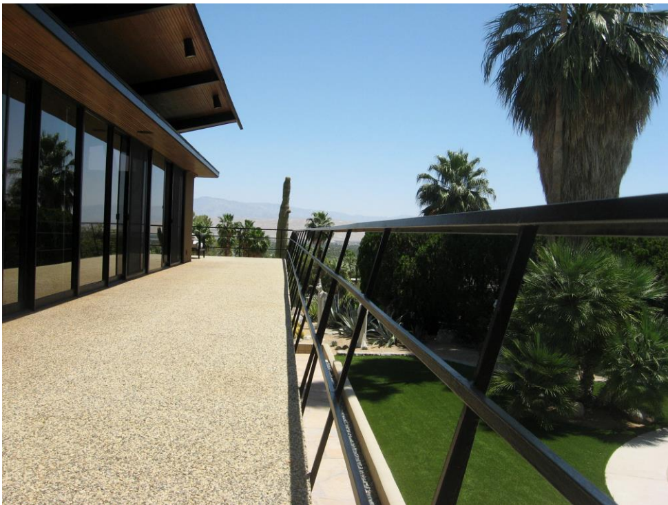
Photo 14: Looking eastwards down balcony. Note the 15-degree tilt of the railing, designed to emulate the structural V-bents. (Author Photo. May 2020)
