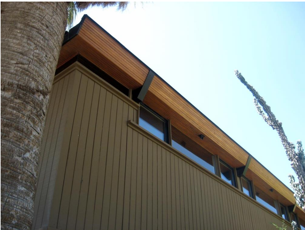
Photo 18: North elevation detail of curved roof with steel straps. (Author Photo. May 2020)
