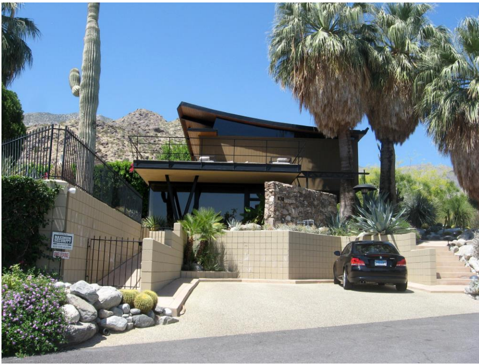
Photo 1: East elevation showing White's 1980s additions including the parking pad and balcony extension. (Author Photo. May 2020)
