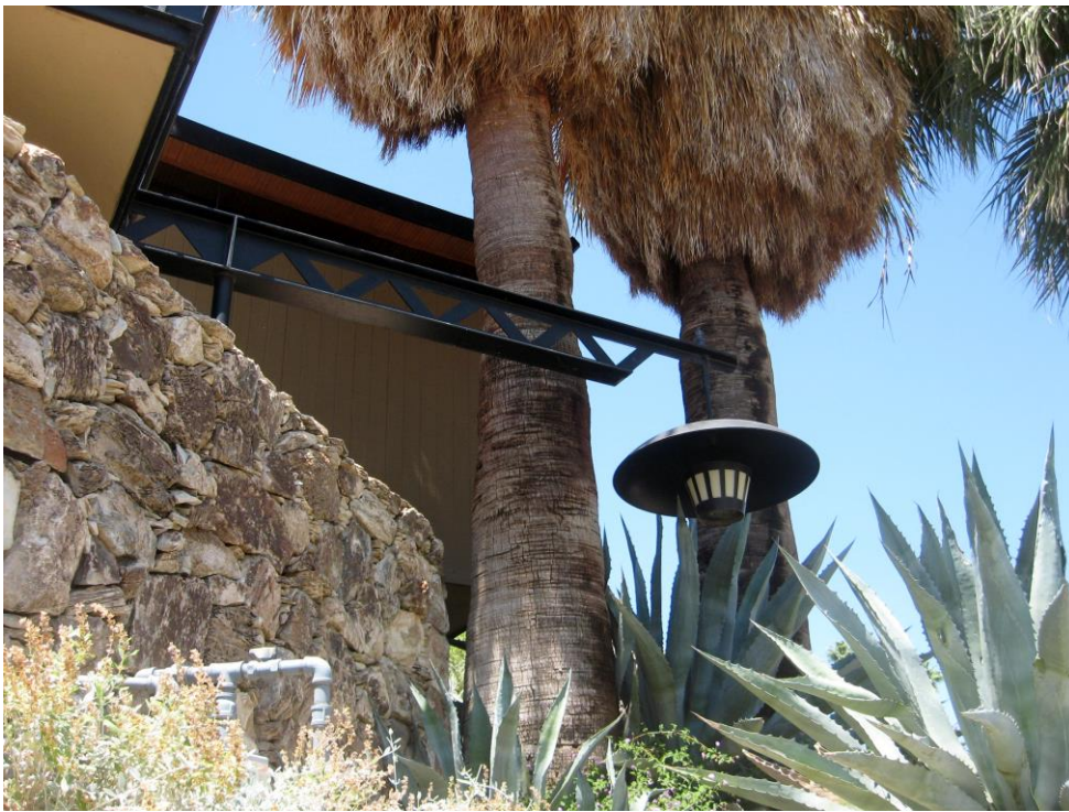
Photo 3: East elevation. Detail of unusual pendant chandelier added by White in the mid-1980s. (Author Photo. May 2020)
