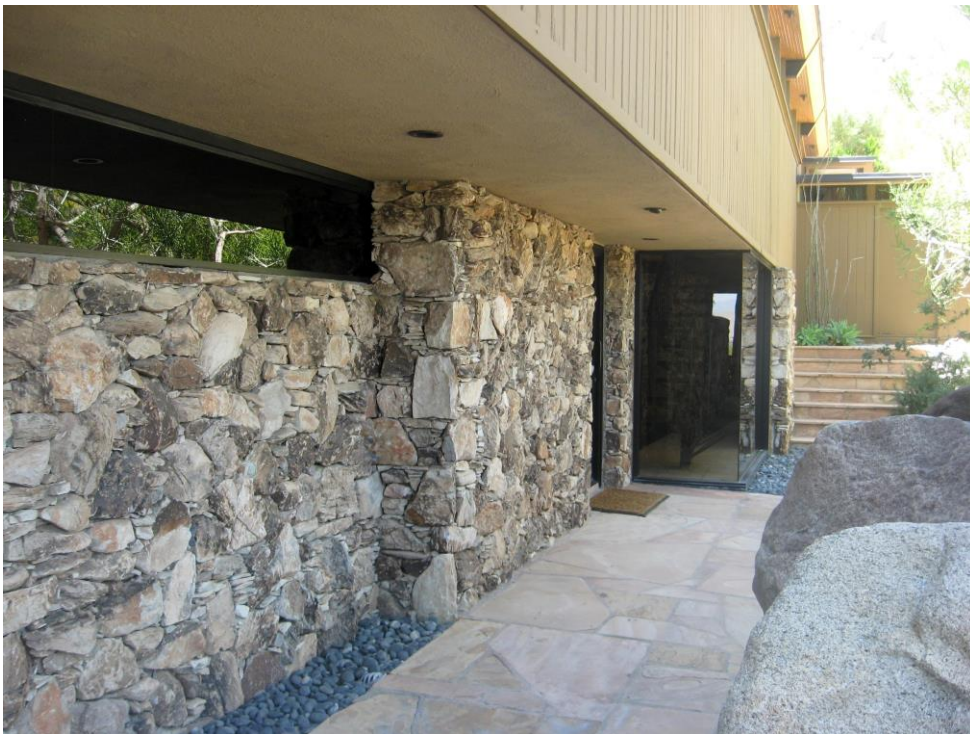
Photo 19: View towards entrance, which was added in 1986. Note Mexican Driftwood used as sheathing. (Author Photo. May 2020)
