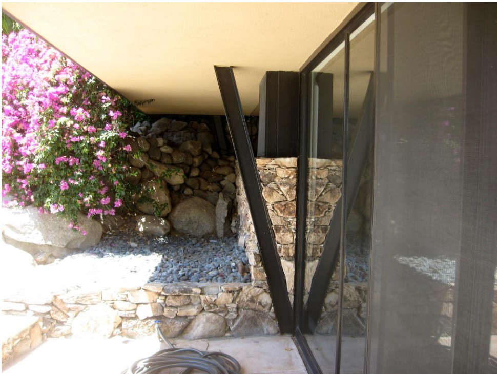
Photo 10: South elevation looking west at Mrs. Alexander's former studio. Note the different combinations of stones. (Author Photo. May 2020)
