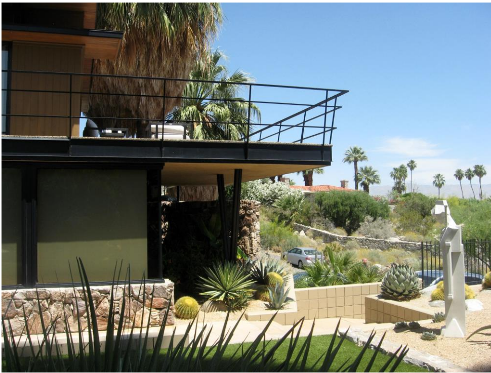
Photo 13: South/east elevation juncture showing balcony extension. Sprite sculpture was designed by Frank Lloyd Wright for Midway Gardens. (Author Photo. May 2020)
