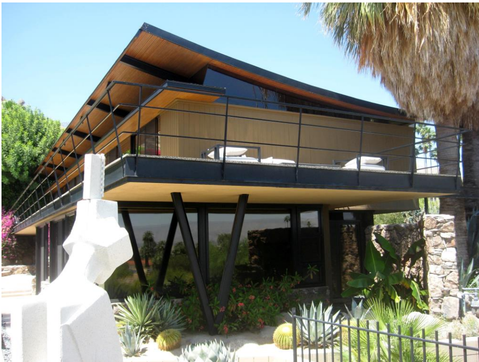
Photo 12: East elevation showing south elevation and White's 1986 additions. (Author Photo. May 2020)
