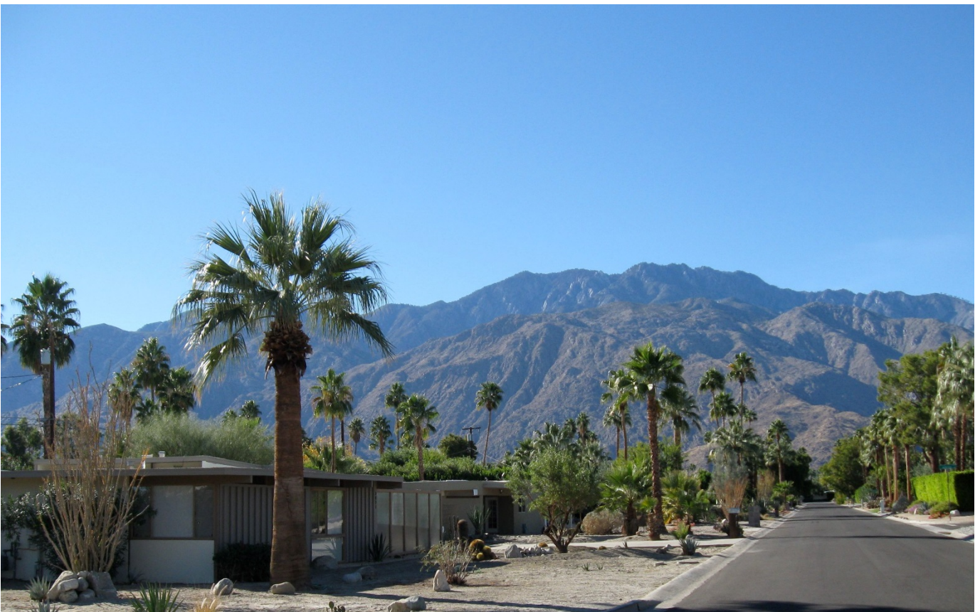
View of front elevation, looking west
