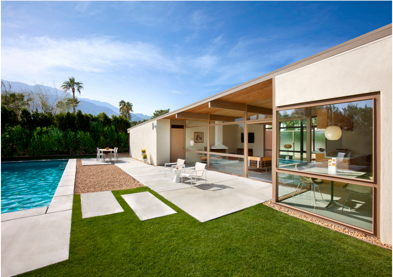
View of rear elevation (without patio cover) looking west
