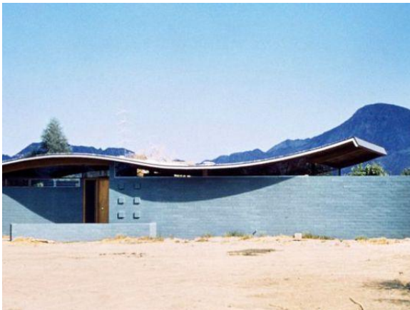
Miles Bates House, Palm Desert 1955. (Photo: Historical Society of Palm Desert/Special to the Desert Sun)
